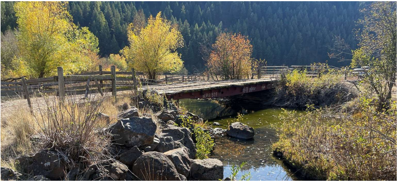
Figure 5-1. Railcar bridge located upstream of Salmon Creek (looking downstream).
