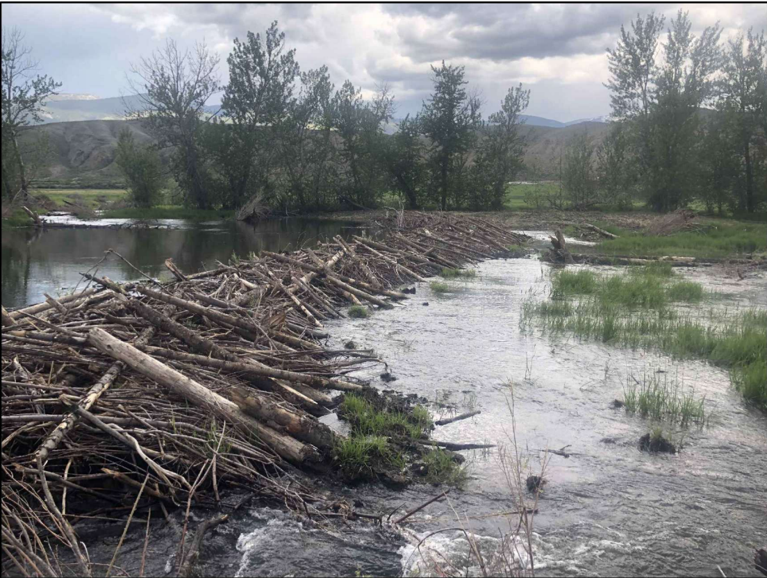
EXAMPLE OF A BEAVER DAM ANALOGUE ON A SIDE CHANNEL OF THE LEMHI RIVER IN IDAHO. PHOTO WAS TAKEN DURING SEASONAL PEAK FLOW IN THE SPRING, FLOW IS LEFT TO RIGHT.
