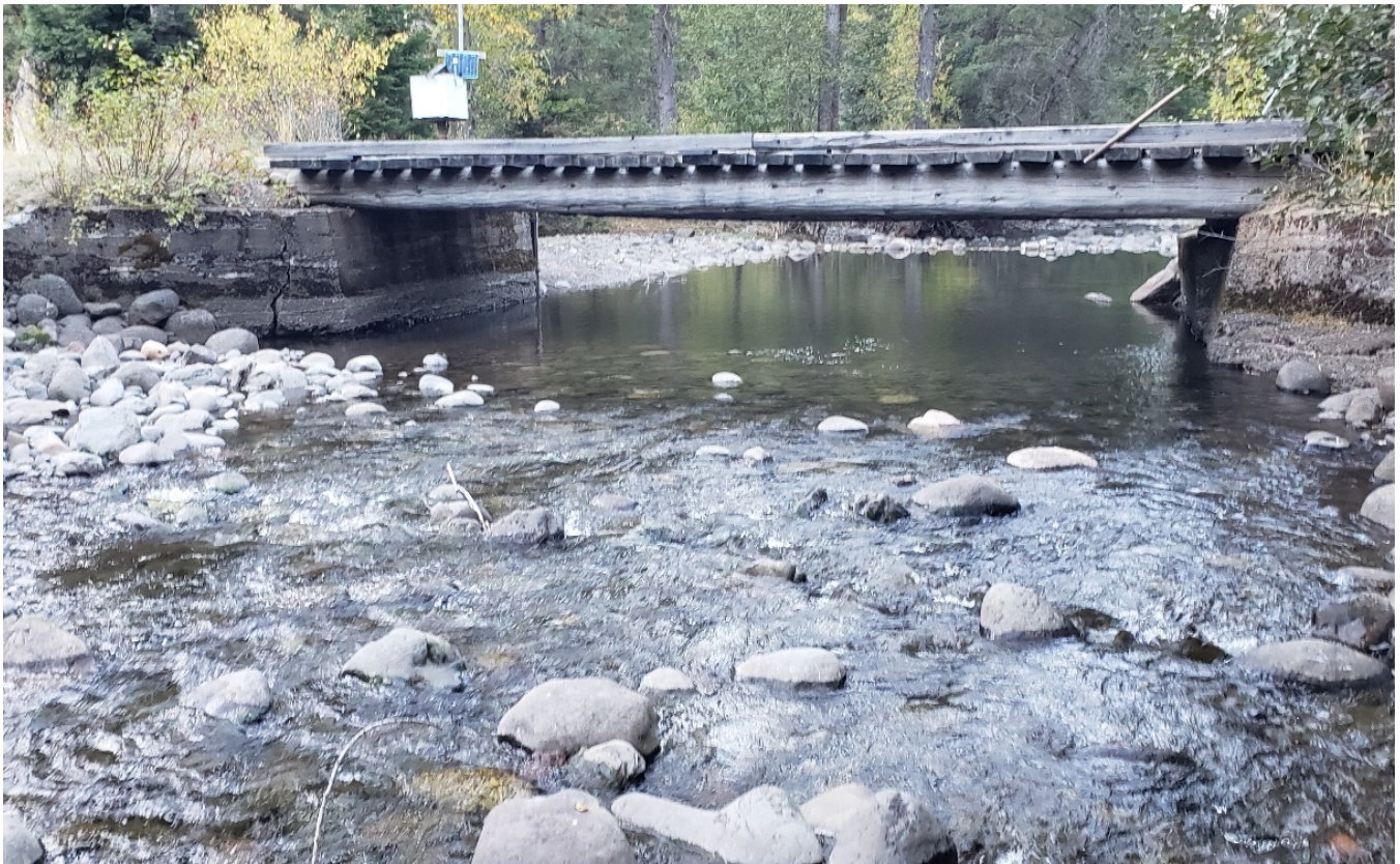
Figure 3-10. The private bridge where the OWRD gage is located at RM 3.3.
