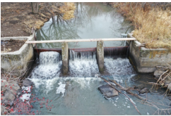
Figure 1. Weaver Diversion (LC5) looking upstream..png
