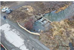
Figure 2. Weaver Diversion (LC5) aerial view from the southwest..png
