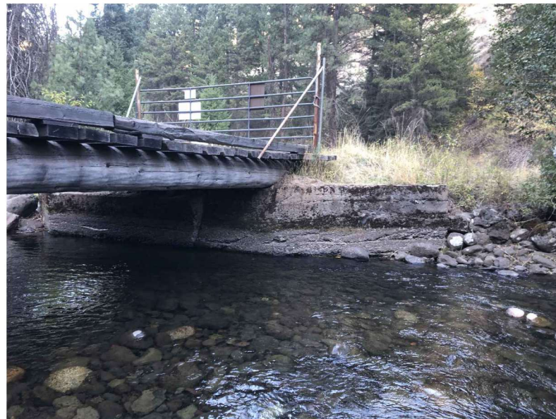
17. PHOTO OF THE EXISTING BRIDGE AT THE DOWNSTREAM END OF THE PROJECT REACH.
