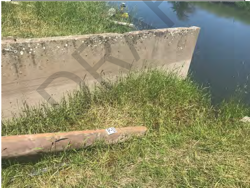
Pump 4 intake and concrete wall, facing upstream (Previously referenced as Pump 11)
