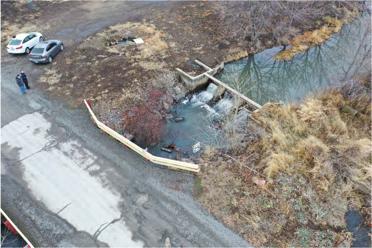
Photo 2: Looking at LC5 from the southwest.
