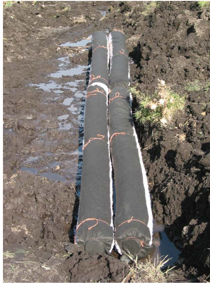
TYPICAL COLLECTOR INSTALLATION
