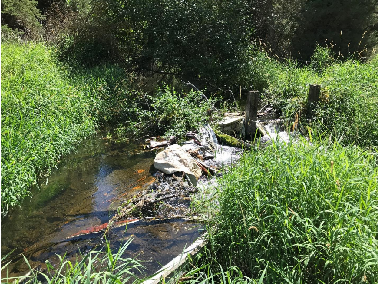
Diversion structure – photo taken on August 22, 2019
