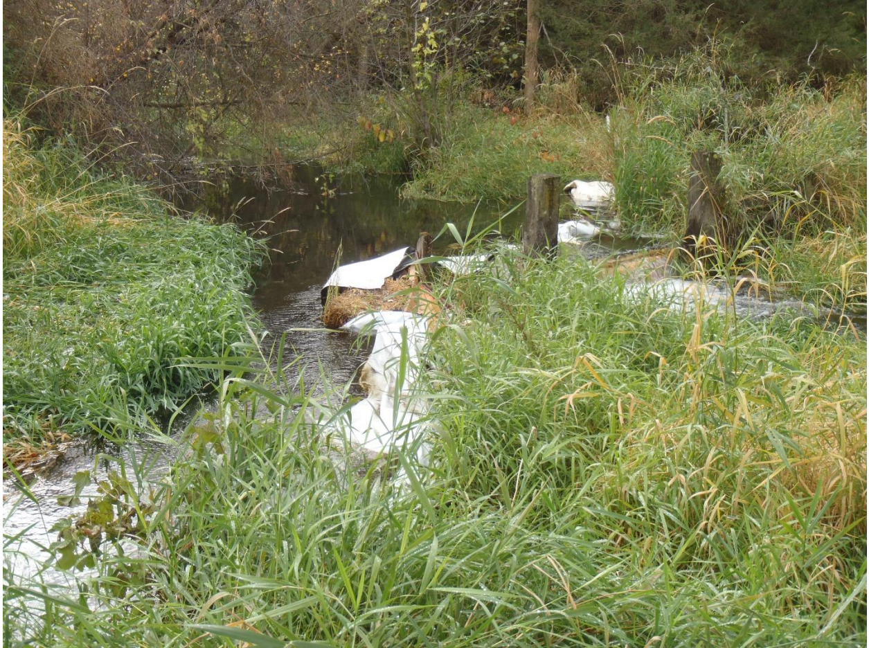
Diversion structure- photo taken October 17, 2016
