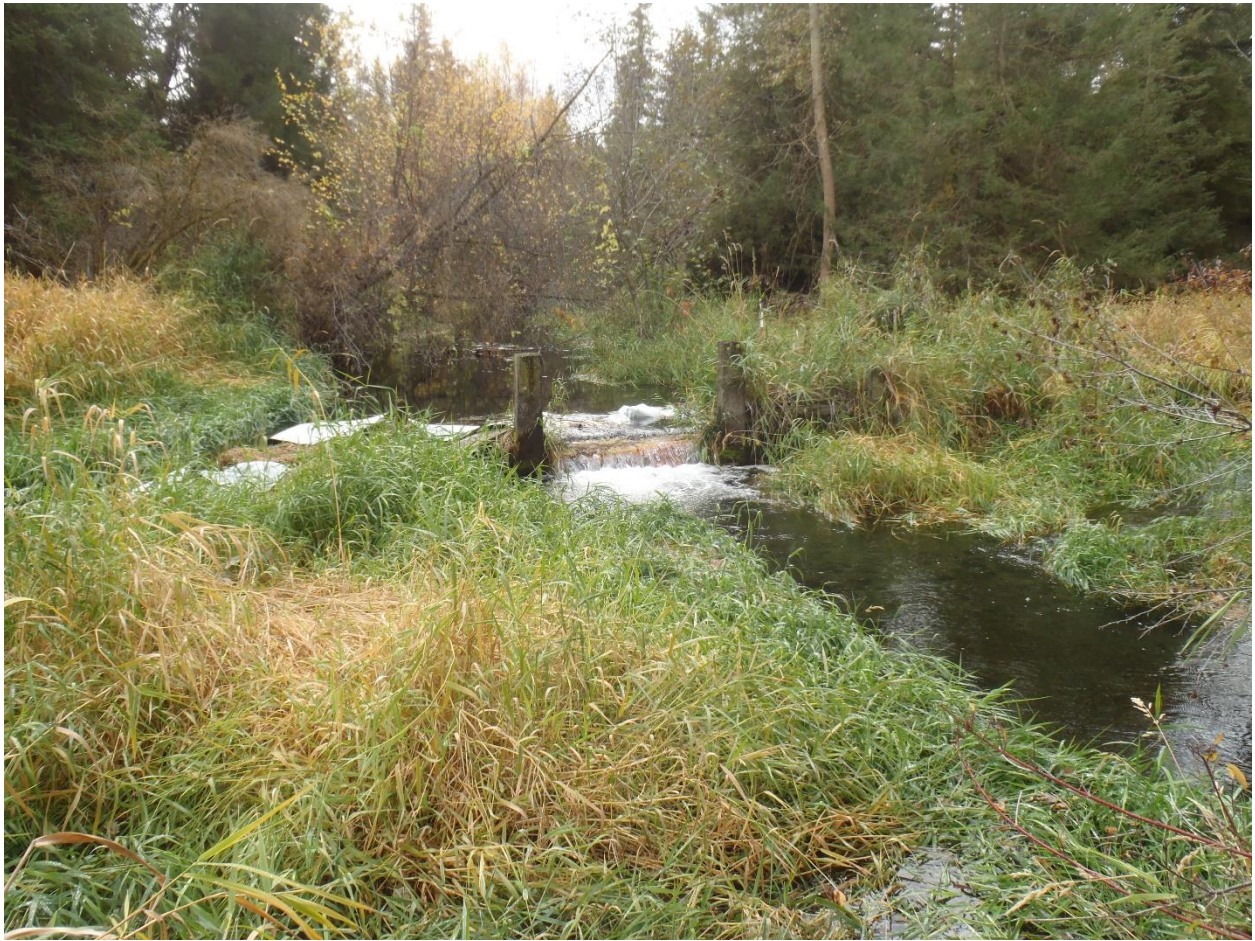
Diversion structure- photo taken October 17, 2016
