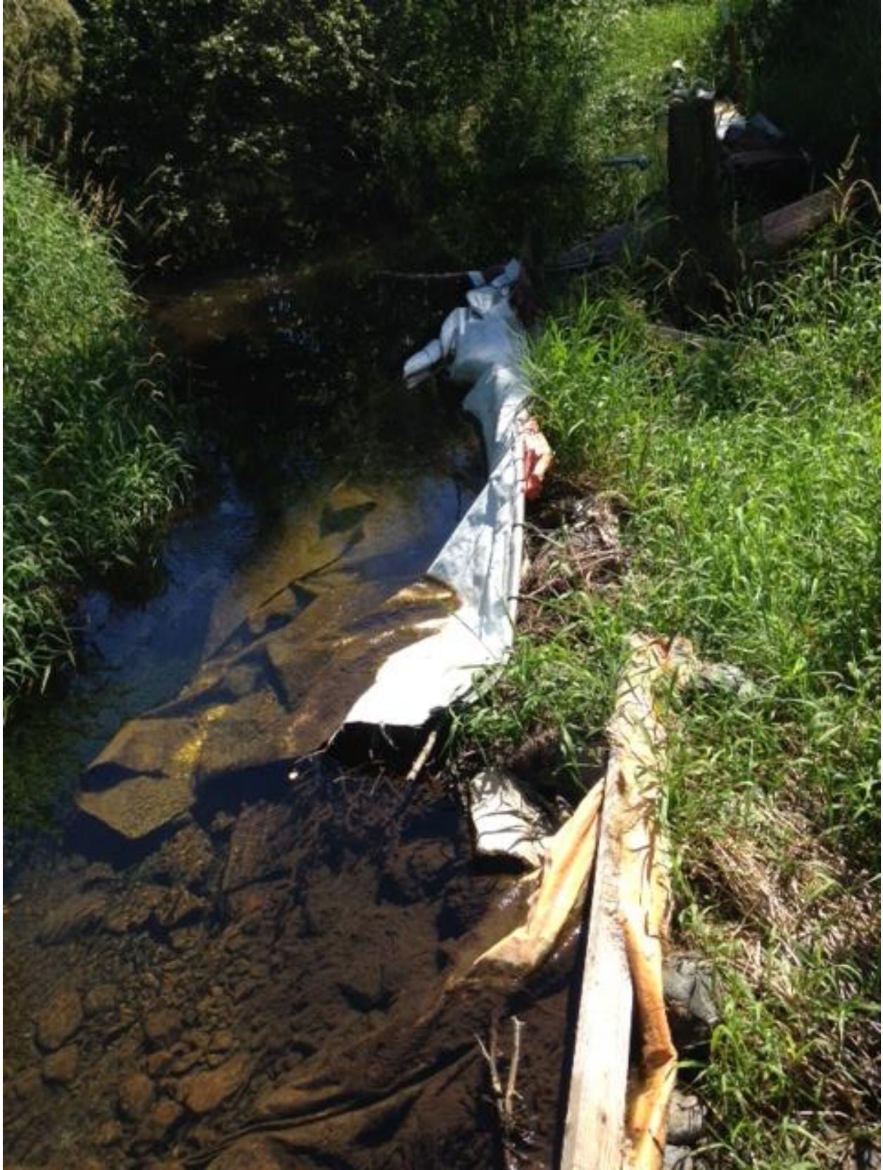
Diversion structure- photo taken July 30, 2015
