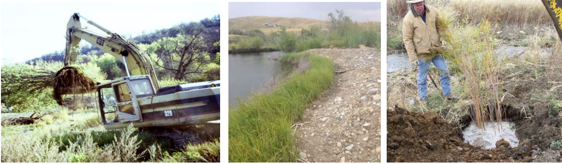
Figure 14. From left to right various planting techniques– willow clump planting (Hoag, 2003), wetland sod mats (2021), cluster planting (Hoag, 2009).
