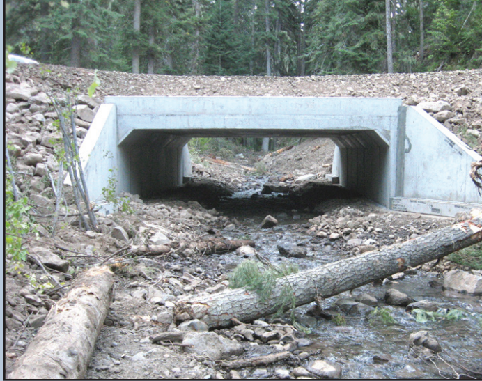
Photo 5: Post-project photograph taken from same location as photo 2. The crossing has been replaced with a concrete structure, and the log weir has been removed. Thirteen steps have been installed and are mostly subsurface features to maintain channel grade and elevation. This structure is much wider than the previous arch and is able to pass debris as it flows downstream, eliminating the need for a trash rack.
