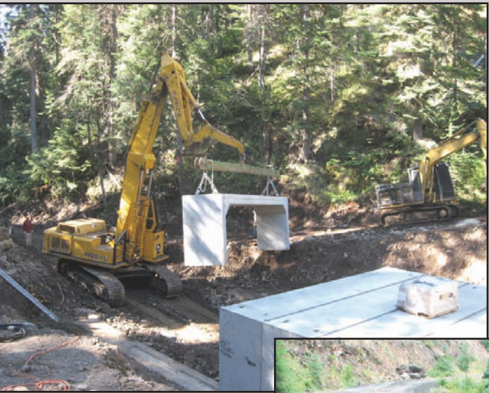
Photo 7: Deer Creek has been diverted around the work site, the arch has been removed, and the footings have been excavated and are in the process of being formed and poured on-site. When re-routed, Deer Creek will flow between the two footings in the photo.
