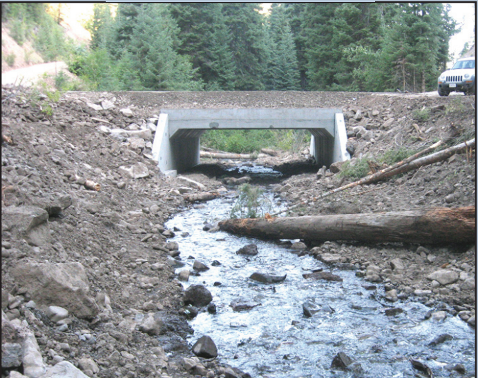
Photo 3: Looking down at the new crossing. Fish passage conditions have been greatly improved, and the placement of logs and other woody material enhances habitat conditions in the construction area.
