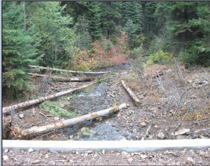
Photo 4: Standing on top of the new crossing looking downstream. Vegetation has been planted, logs have been placed to improve habitat, artificial barriers have been removed, and the risk of the crossing to fail has been greatly reduced.
