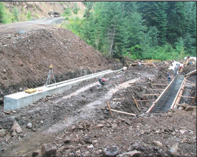
Photo 7: Deer Creek has been diverted around the work site, the arch has been removed, and the footings have been excavated and are in the process of being formed and poured on-site. When re-routed, Deer Creek will flow between the two footings in the photo.
