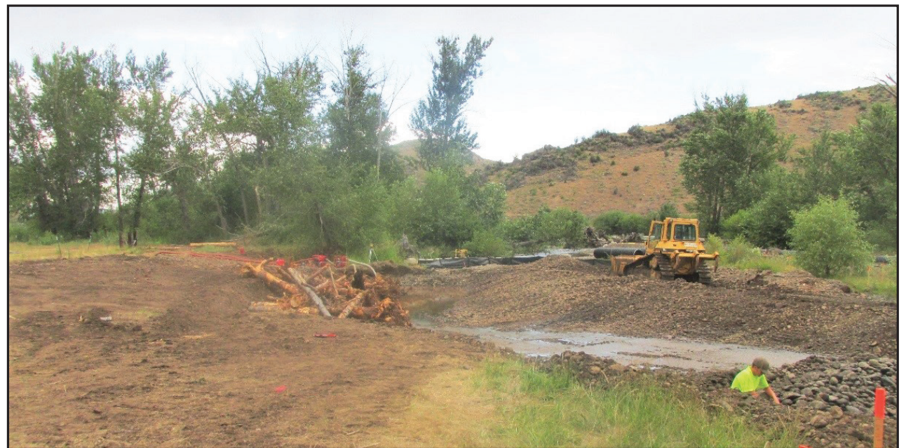
Above: Construction occurs on the lower end of the project, including large wood placement and channel regrade. The main flow of Catherine Creek has to be diverted for this component to take place. (Photo: ODFW)
