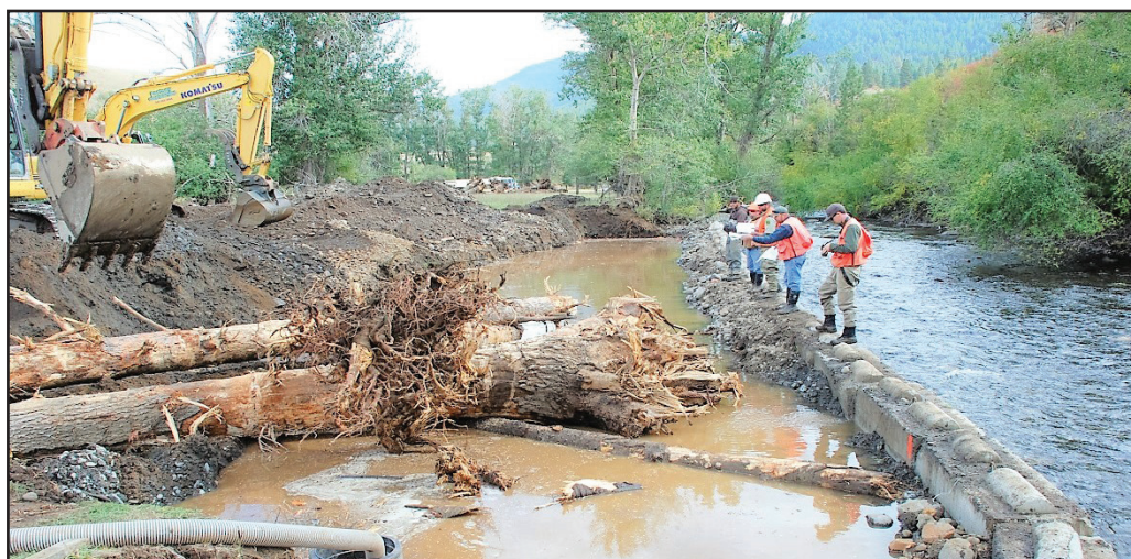
Above: Construction of a fish habitat structure in an isolated work area on Catherine Creek, 2014. (Photo: ODFW)
