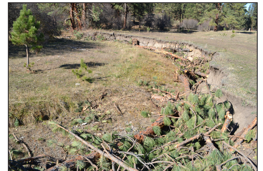
ABOVE: Graves Creek in October 2013 after project implementation. These structures will stabilize actively eroding streambanks and provide habitat complexity and diversity.
