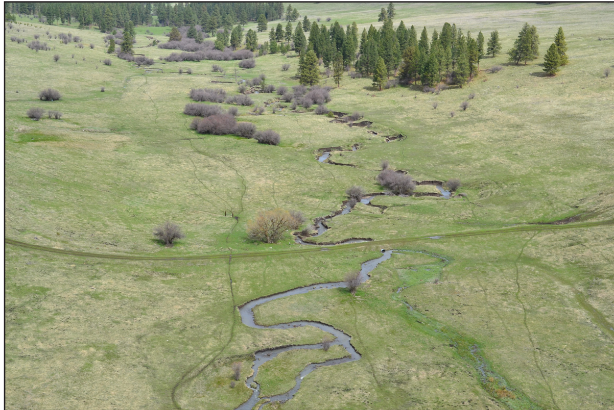
ABOVE: April 2013 image of Graves Creek. Showing limited riparian vegetation, entrenched cut banks, and abandoned historic side channels. (Before restoration)
