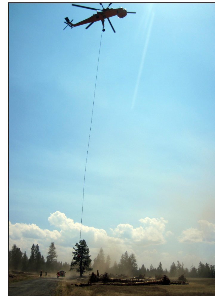
ABOVE: A helicopter picking up rootwads for transport to the Meadow Creek project site for installation. Photo by USFS.
