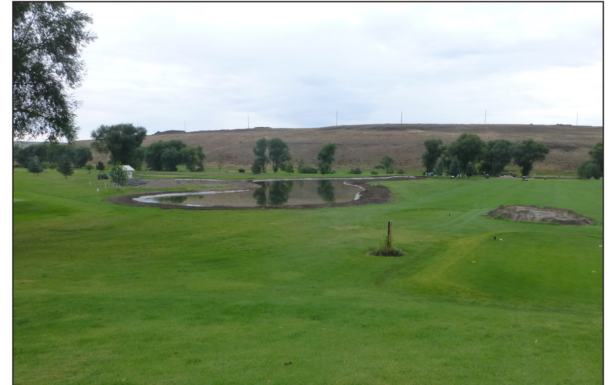
ABOVE: This photo taken from the same location as the photo in the middle of page 4 shows the completed and operational storage pond and pump station. The bare ground border around the pond will be landscaped in spring 2014
