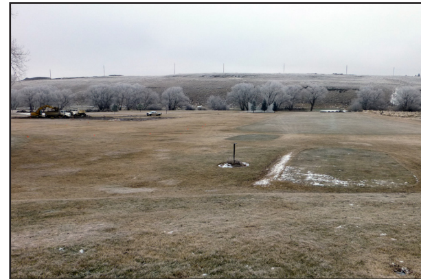
ABOVE: This photo was taken on the first day of pond construction on January 3, 2013. The COE wastewater mainline runs along the toe of the hill in the background. The storage pond and pump house will be installed in the foreground.
