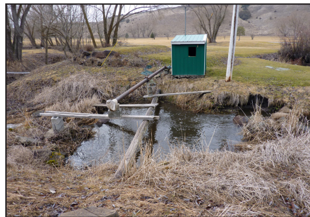
ABOVE: The removed golf course pump station. Notice how the pool above the dam has widened the creek channel and is causing erosion under the power pole and pump house.
