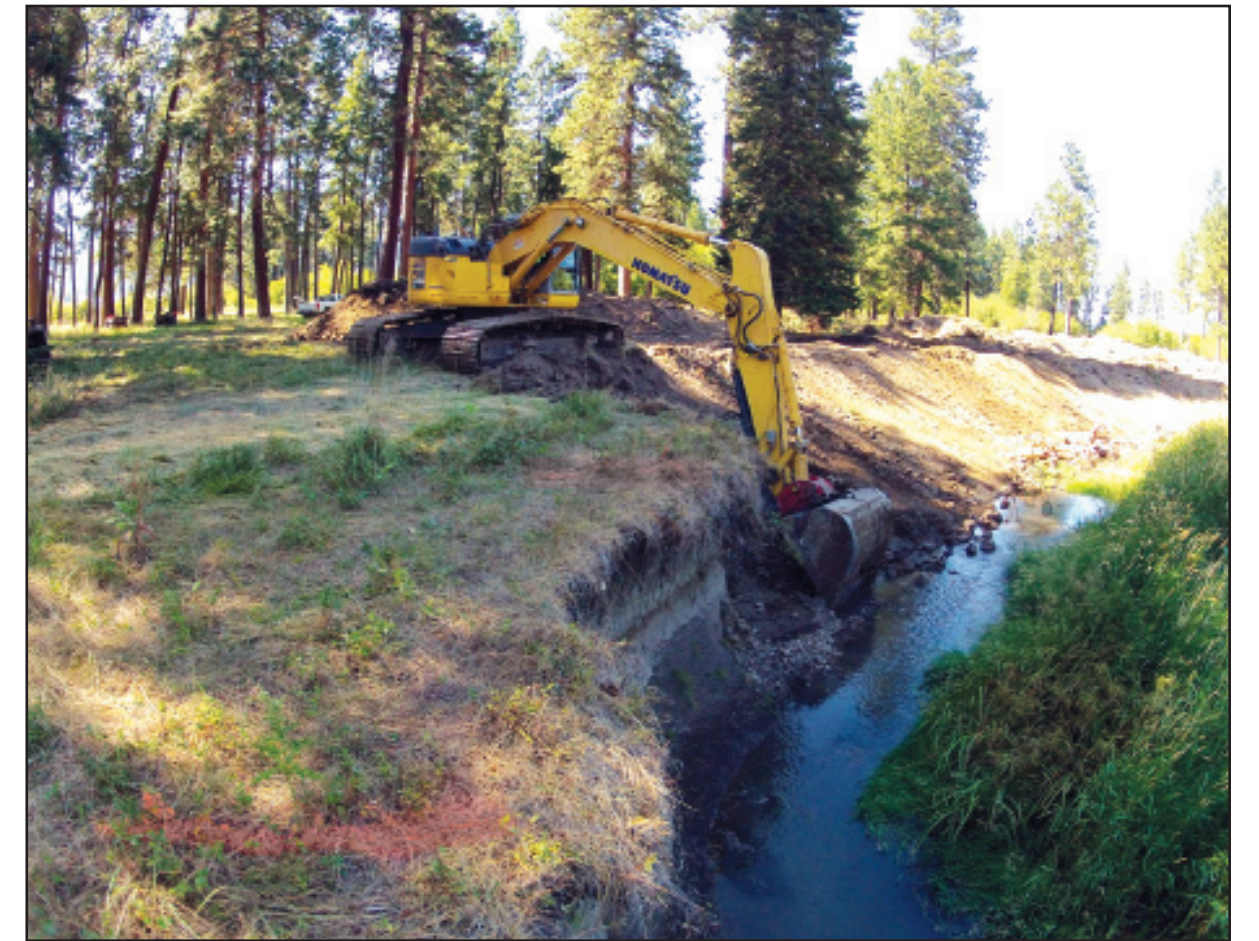
This photo was taken during construction of the Willow Creek Restoration and Enhancement Project. The image shows the re-contouring of the stream bank, which was extremely eroded and vertical in some areas. Large wood structures also were placed in this area of the project.
