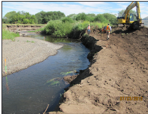
ABOVE: Vertical Banks prior to construction re-sloping and setback.
