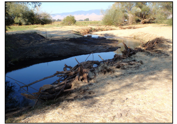
ABOVE: New meander. Excavated and re-sloped banks and widened floodplain. Large wood structures placed. Banks were mulched, re-seeded, and planted.
