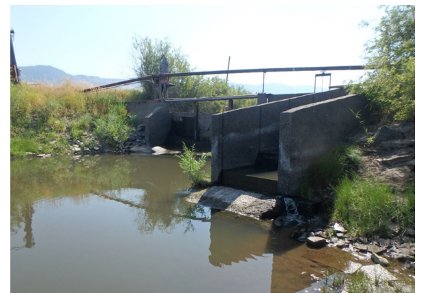
The Elmer Dam fish ladder entrance showing inadequate flow for passage during summer conditions. (Courtesy of Jim Webster)
