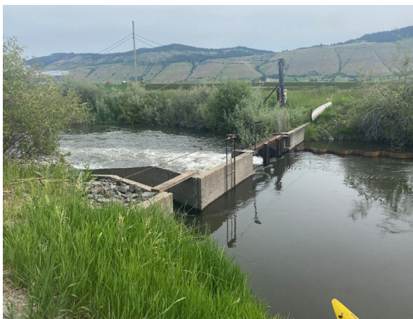
The Elmer Dam and fish ladder prior to construction. (Courtesy of Jim Webster)
