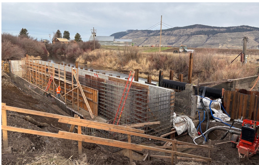
Forming construction for a new fishway at Elmer Dam.
