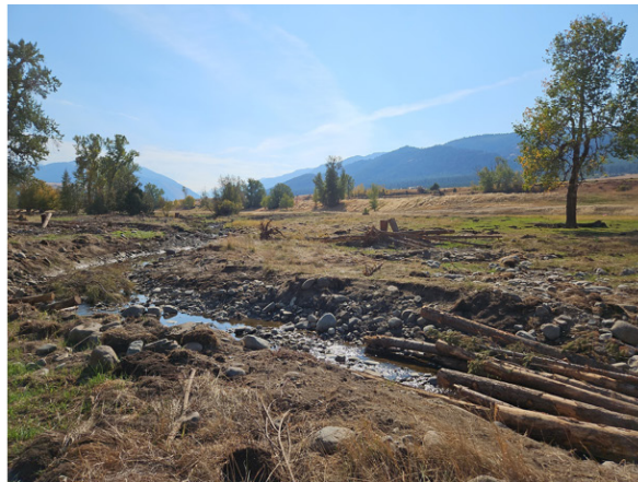
Before and after construction of secondary channels designed to enhance habitat and natural flow patterns. (Courtesy of the Nez Perce Tribe)
