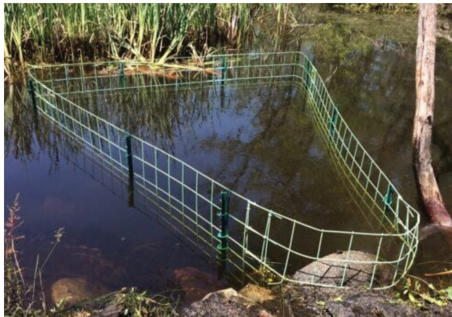
Example of a keystone culvert. (Photo courtesy of The Beaver Institute)
