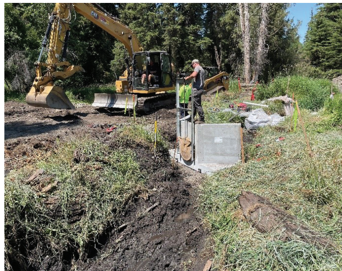
LEFT: ODFW staff oversee riffle construction that replaced the irrigation diversion structure. RIGHT: Post-setting the new headgate. (Photos courtesy of ODFW)
