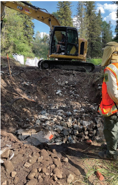
LEFT: ODFW staff oversee riffle construction that replaced the irrigation diversion structure. RIGHT: Post-setting the new headgate. (Photos courtesy of ODFW)
