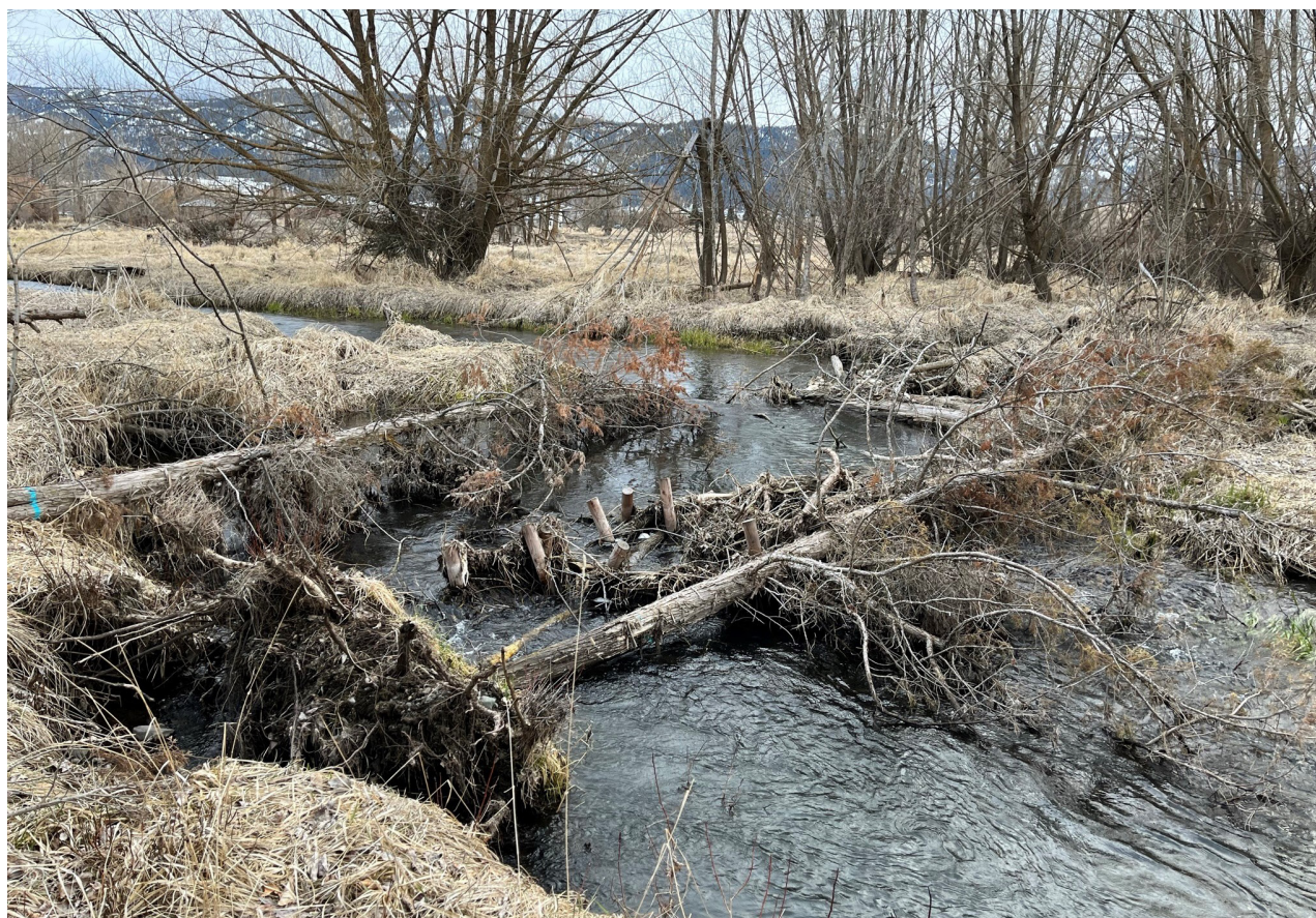
Small juniper trees used in conjunction with a post-assisted log structure in a side channel create overhead cover for juvenile life stages of salmon and steelhead as well as adult holding cover. Photo by Ian Wilson, GRMW.
