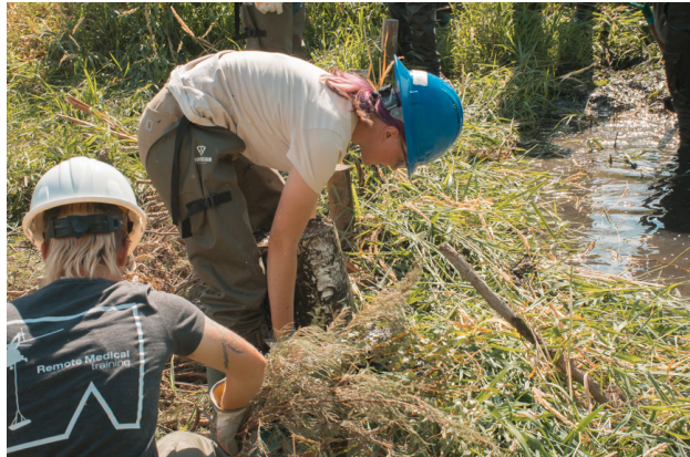
Isabel Mcguire, a junior at Wallowa High School, dumps a bucket of mud collected from the river bank on top of the beaver dam analog. (courtesy of Avery Stanton)
