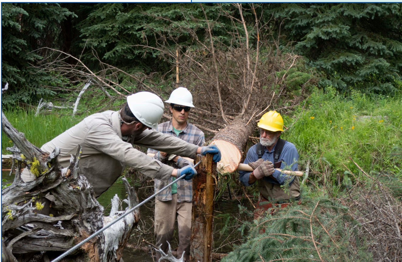
U.S. Veterans work a griphoist and other hand tools to place a piece of large woody debris into the stream. (Photo: Levi Old)
