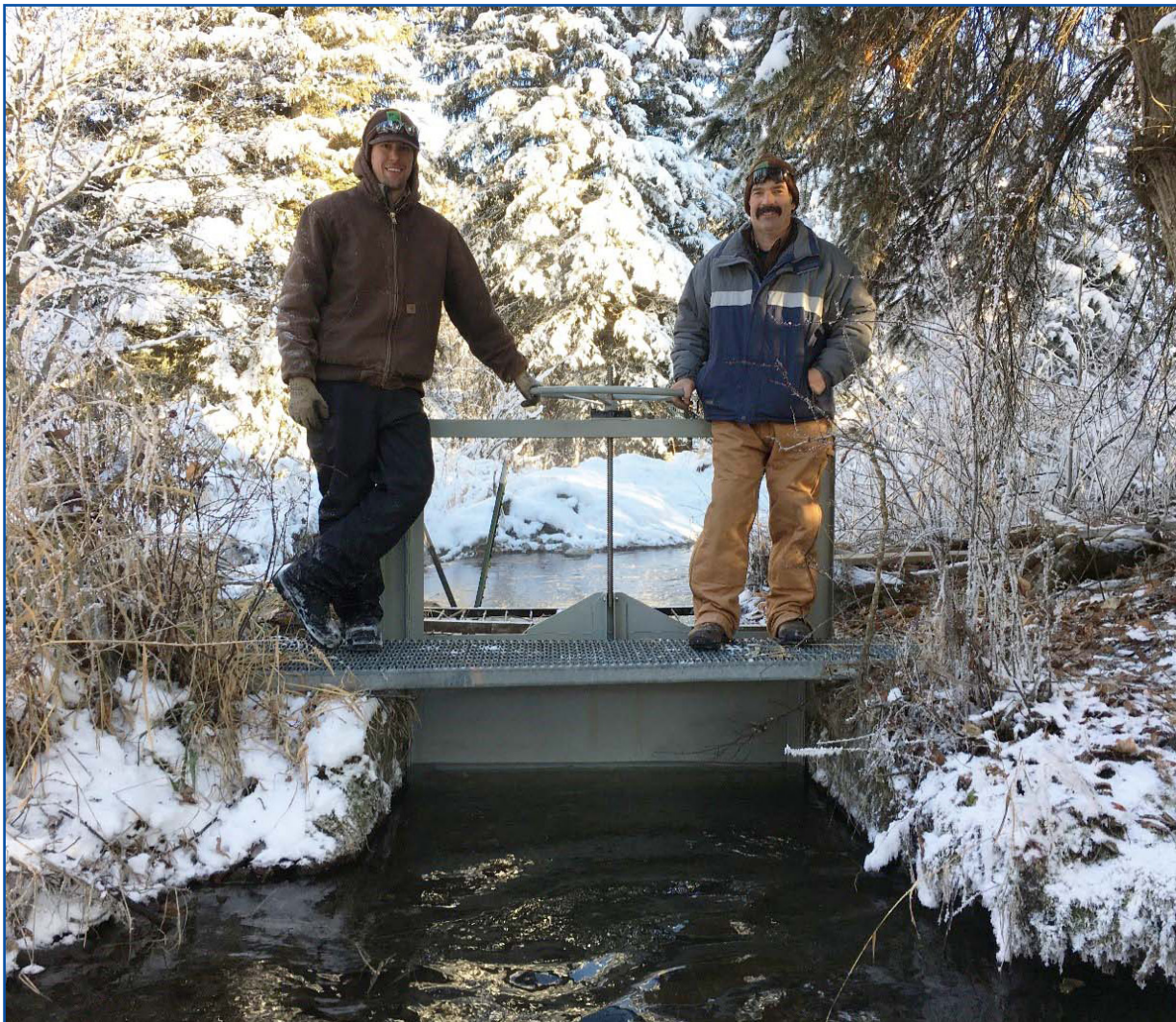
Chuck (right) with another ODFW employee, Chad (left) at the newly installed headgate. (Photo: David Bates)
