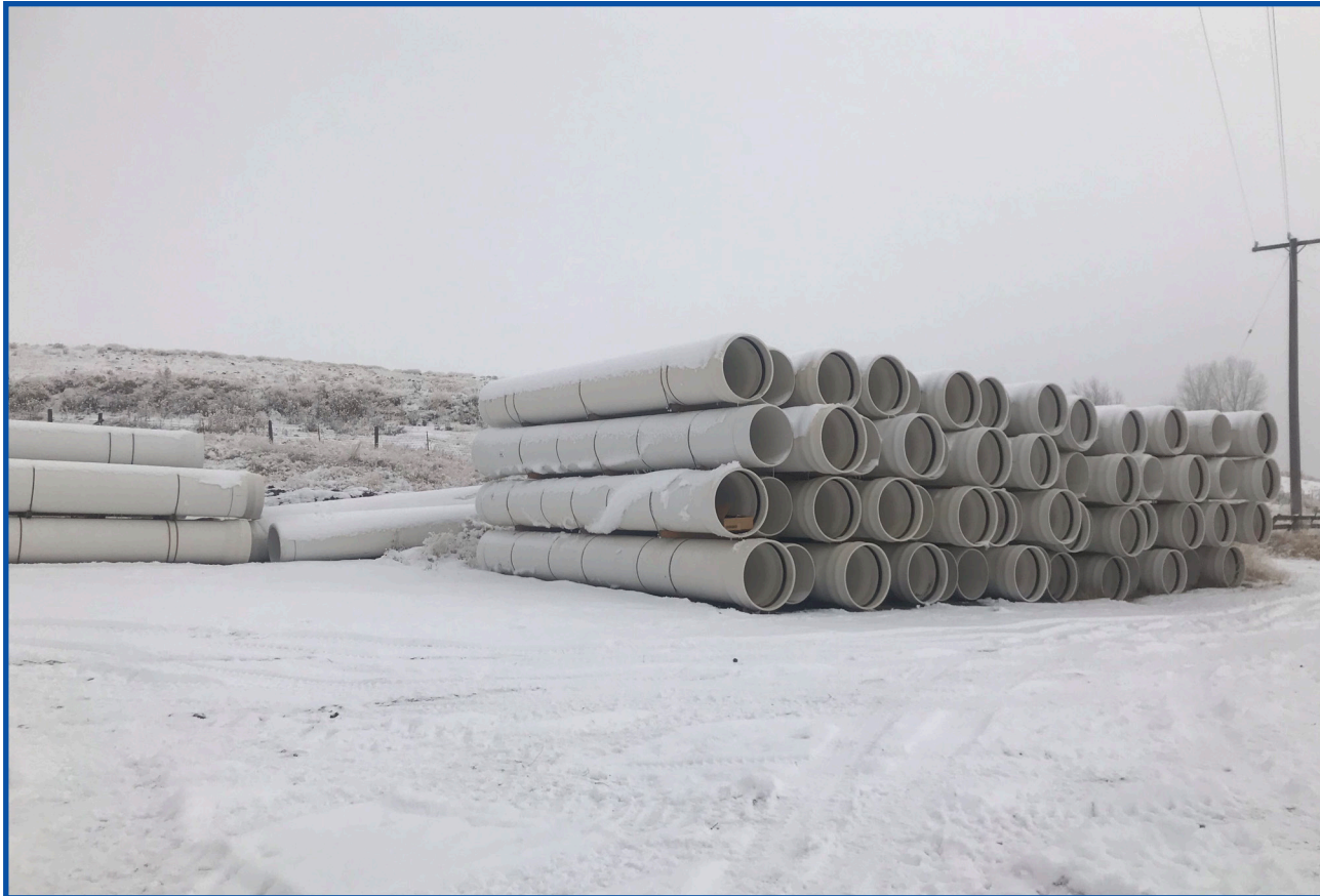
Sections of pipe at a staging area waiting to be installed. These sections will help complete phase one of the pipeline, which will stretch approximately five miles. (courtesy of GRMW).
