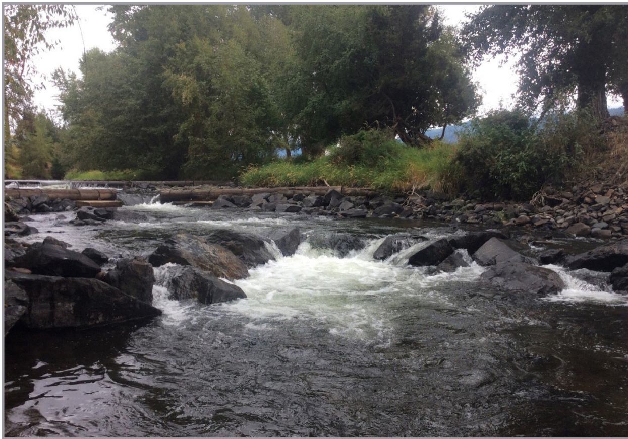
Above: The Tulley Hill diversion structure on the Lostine River before restoration. The diversion is composed of rock and log weirs which have created a velocity barrier for juvenile fish at high flow (courtesy of Katie Frenyea).
