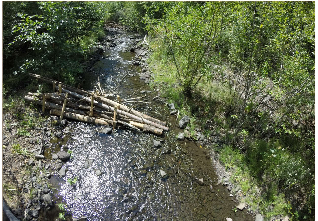
Figure 1. A post assisted log structure (PALS) on the South Fork of Asotin Creek immediately after construction. The goal of this structure is to deflect the majority water to one side during high flows, ultimately scouring a pool, creating bars, and providing fast water and predation refuge for steelhead.
