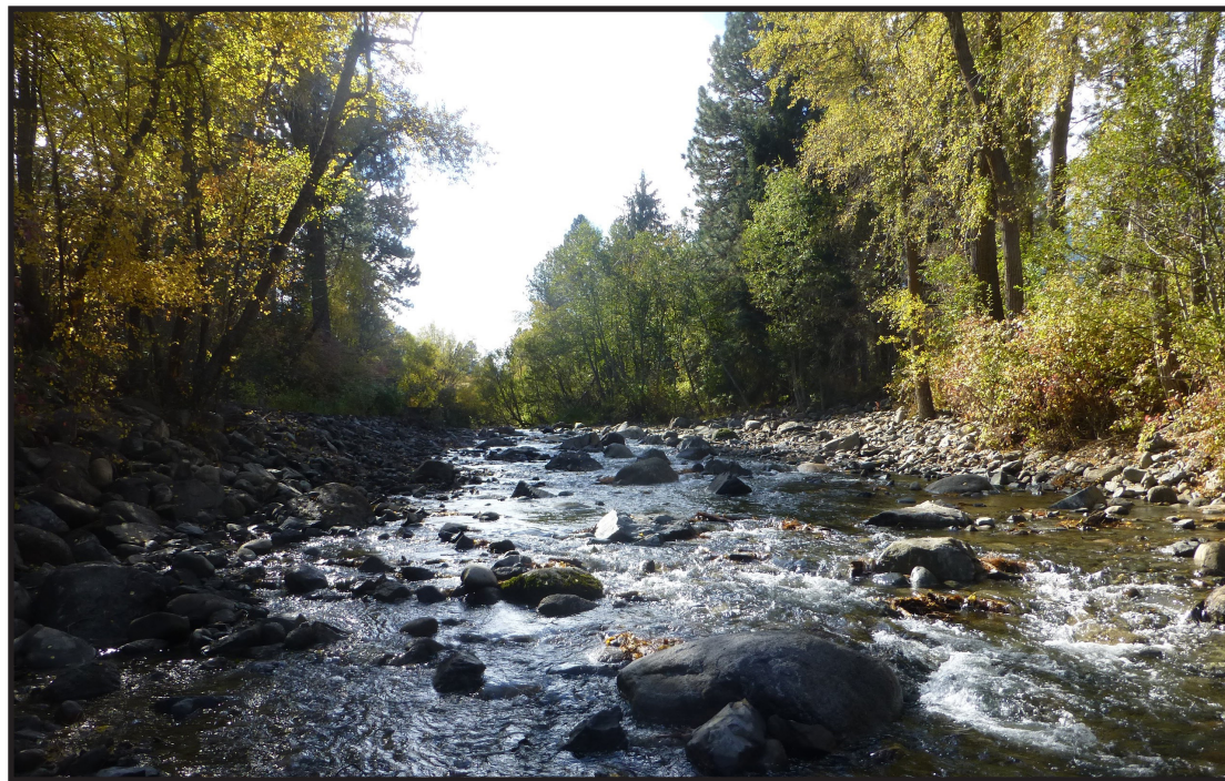
Looking upstream following project completion. The old concrete fishway left intact was overtopped with an engineered roughened channel.
