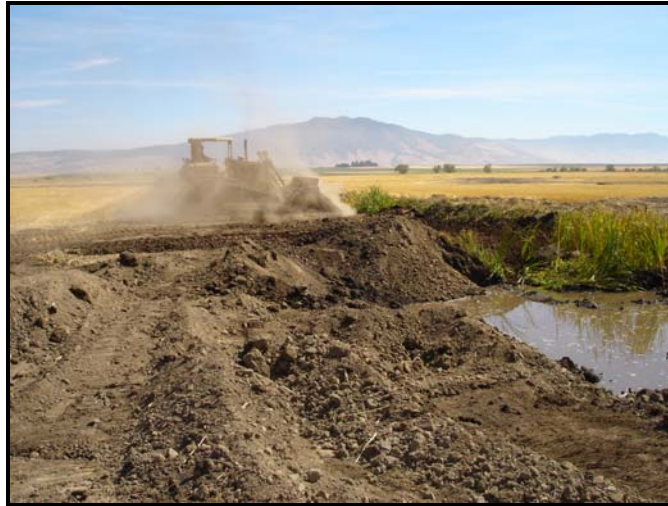
Reclamation of channelized End Creek following activation of restoration channel.
