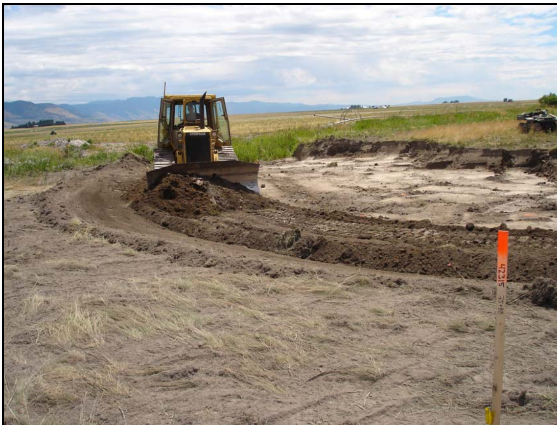
Initiation of channel construction on lower End Creek.
