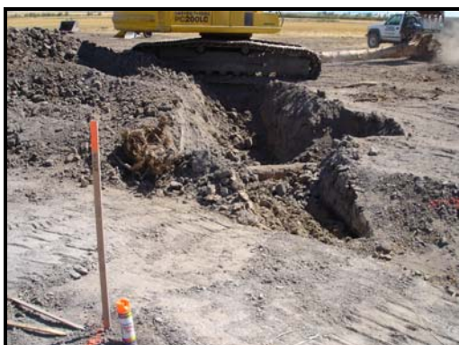
Rootwad revetment installation. Photo illustrates installed footer log and keyway for rootwad and tree bole installation.
