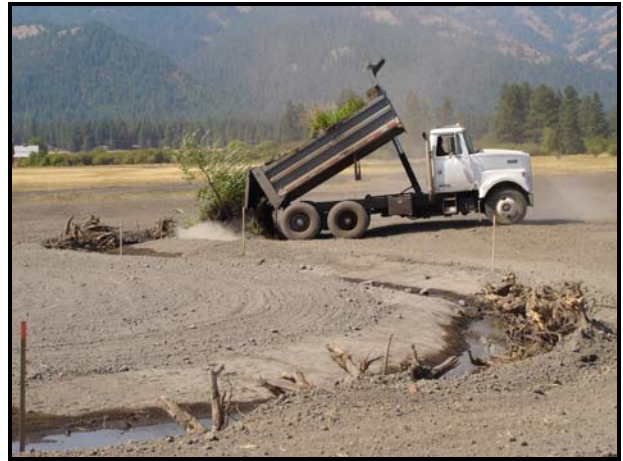
Dump truck hauling and stockpiling plant materials at selected locations along End Creek restoration channel.
