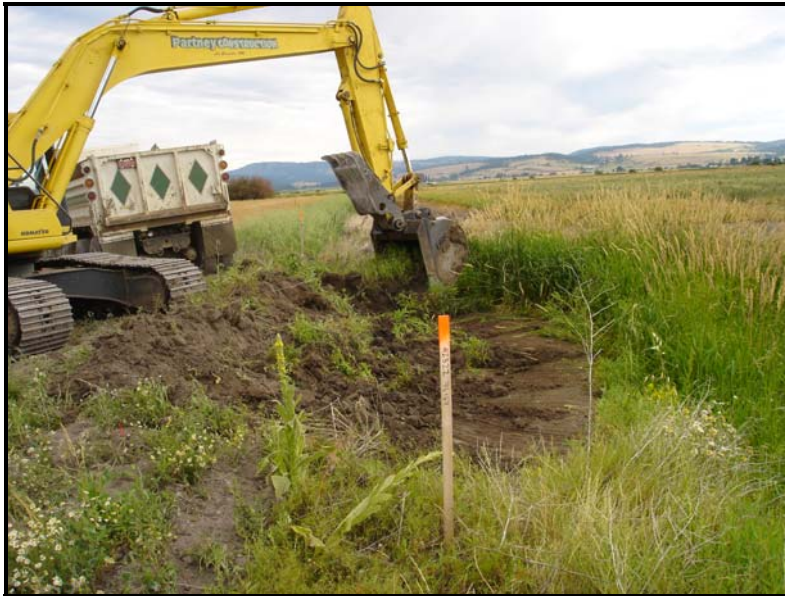
Initiation of End Creek restoration channel construction
