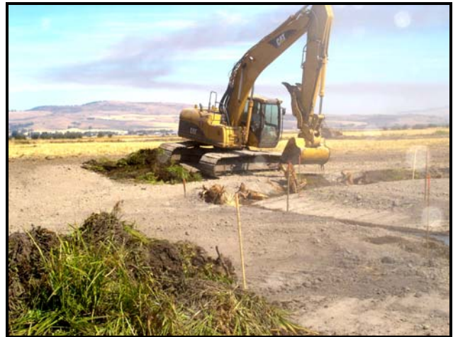
Excavator installing sedge/rush matts along outside stream meander on rootwad revetment
