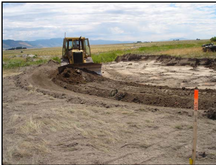
D5 Dozer grading material from floodplain in preparation for bankfull channel excavation by track-hoe
