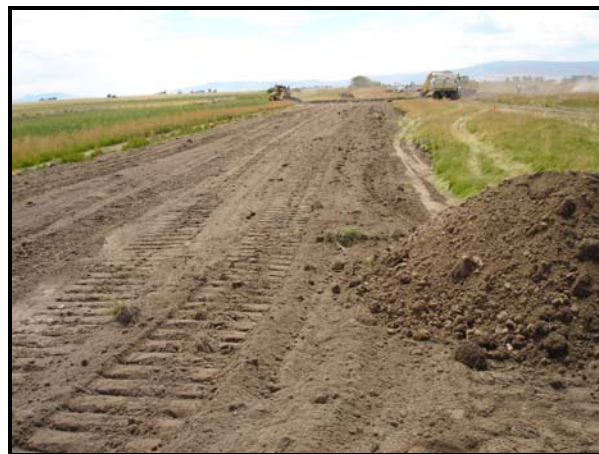
Earthen terrace constructed along eastern project boundary to minimize potential for flooding on adjacent private land
