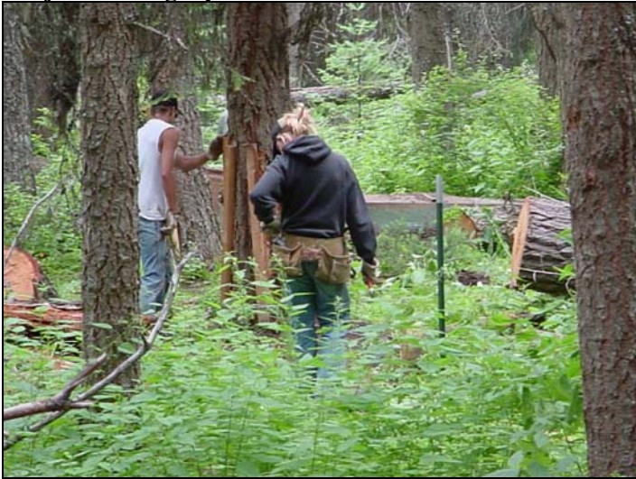
TEC youth crew building fence at Huckleberry spring.
