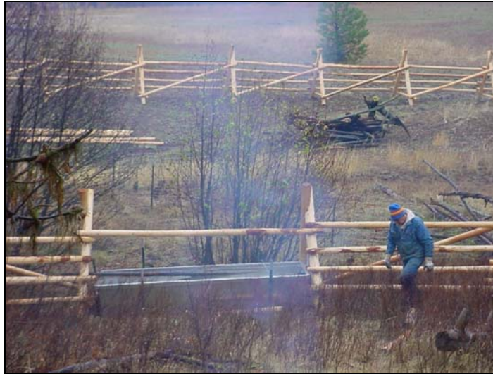
New trough and buck & pole fence at Dougherty spring.
