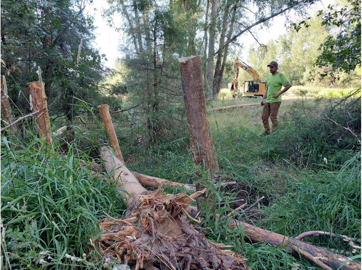
Figure 5. Completed Vertical Post Array in floodplain swale, taken 8/4/22.
