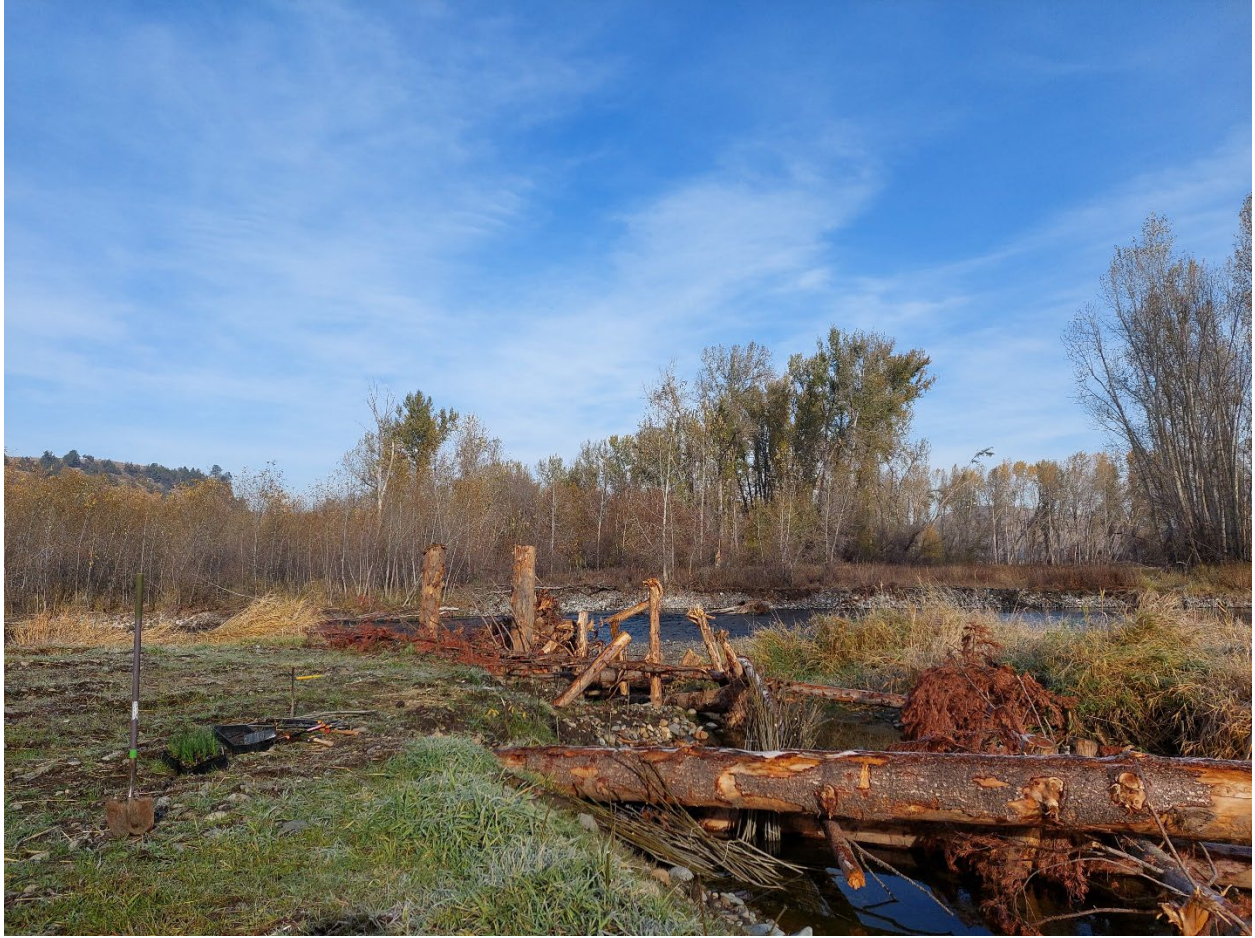
Figure 7. In-progress willow stake and wetland plug planting, taken 10/27/22.
