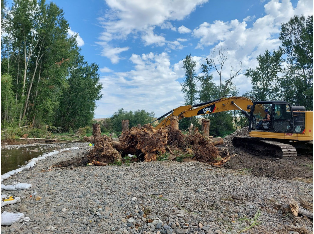
Figure 2. Installation of Large Apex Jam A2, taken on 8/3/22.
