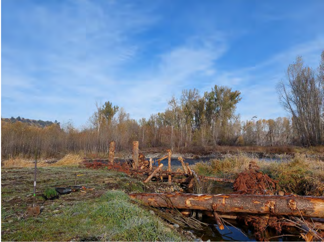
Figure 5. In-progress containerized wetland plug and willow stake planting in Pilot Channel 1-Outlet, taken October 27.
