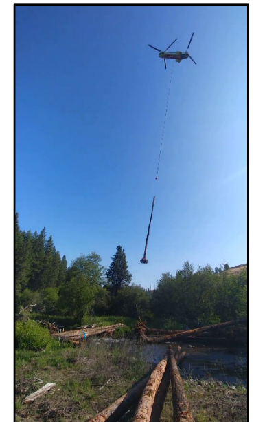
Helicopter placing large wood jam structures
