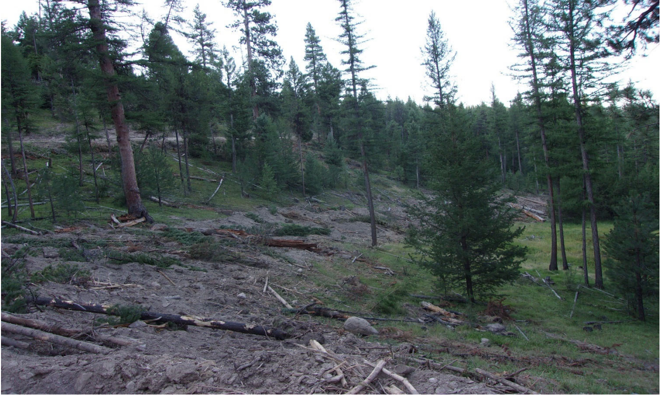
Road Recontour on Access Road to Fly Creek
