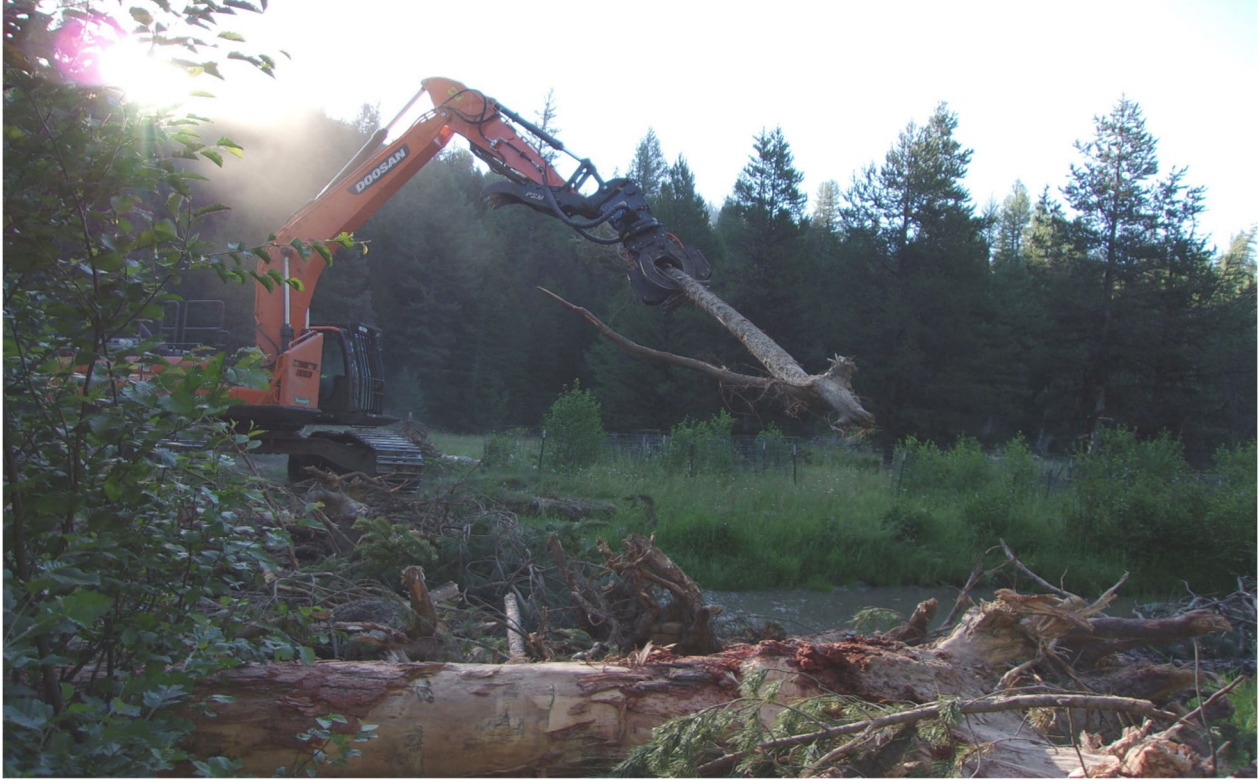
Placement of Wood into Fly Creek
