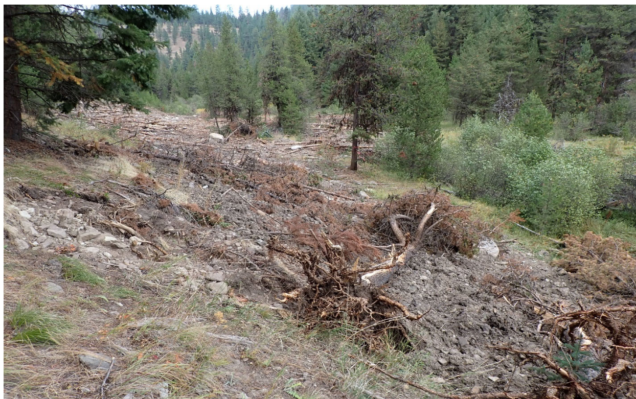
Fly Creek Streambottom Road Recontour
