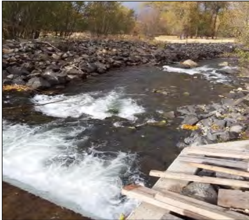
Photograph 4. Existing boulder steps downstream of Poley-Allen diversion sill.
