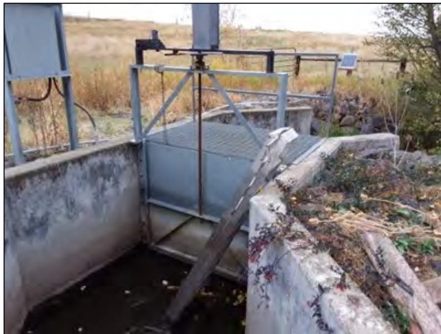
Photograph 2. Existing Poley-Allen irrigation headgate.
