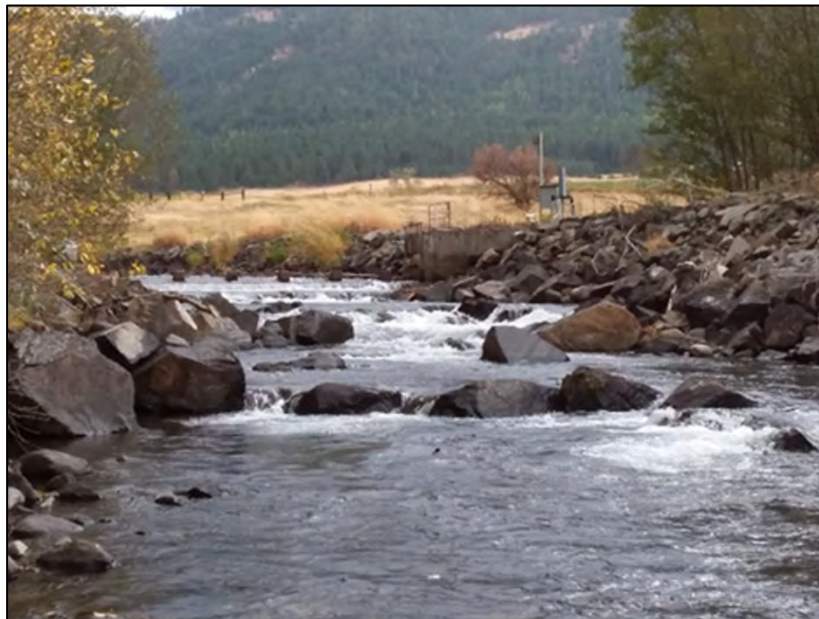
Photograph 5. Existing boulder steps downstream of Poley-Allen diversion sill.
