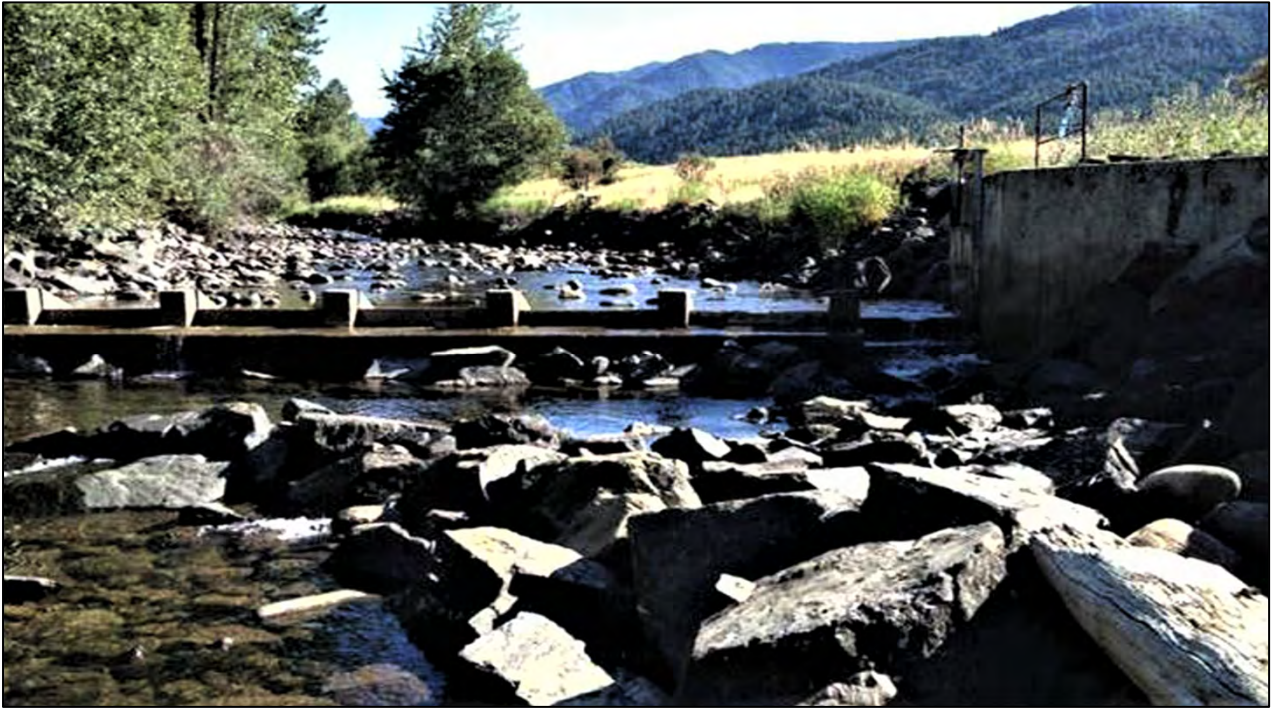
Photograph 6: Upstream reach looking upstream at sill and the plane bed morphology and left-bank channel armoring.
