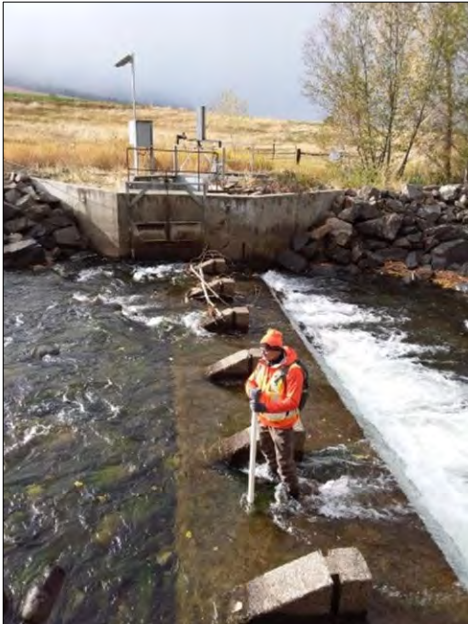
Photograph 3. Existing Poley-Allen diversion sill, irrigation intake, and abutment.
