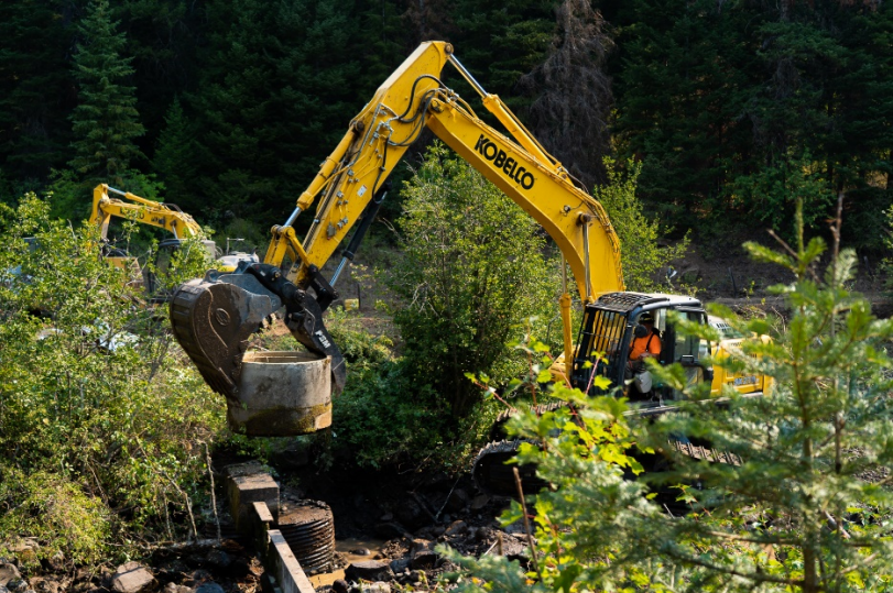
Photo (L & R): Diversion dam removal at middle site on Indian Creek Project.
