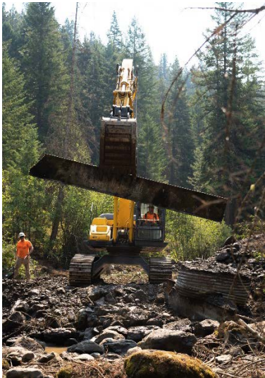
Photo (L & R): Diversion dam removal at middle site on Indian Creek Project.
