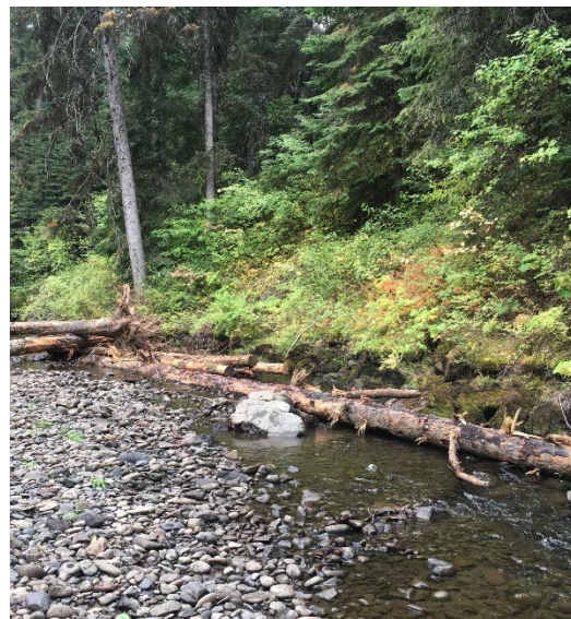
Photo (R): 3-Log LWD Structure - As-Built
