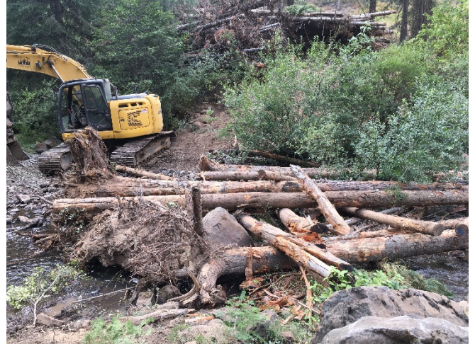
Photo (L): Removal of old culvert and roadbed at the middle site. Photo (R): Deflector LWD Structure at middle project site.
