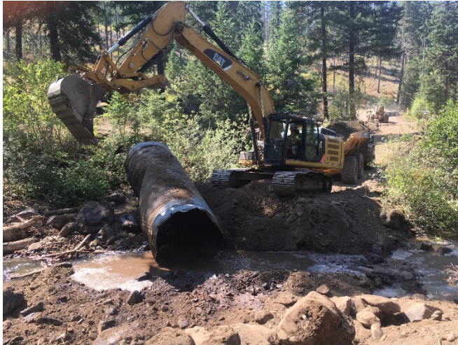
Photo (L): Removal of old culvert and roadbed at the middle site. Photo (R): Deflector LWD Structure at middle project site.
