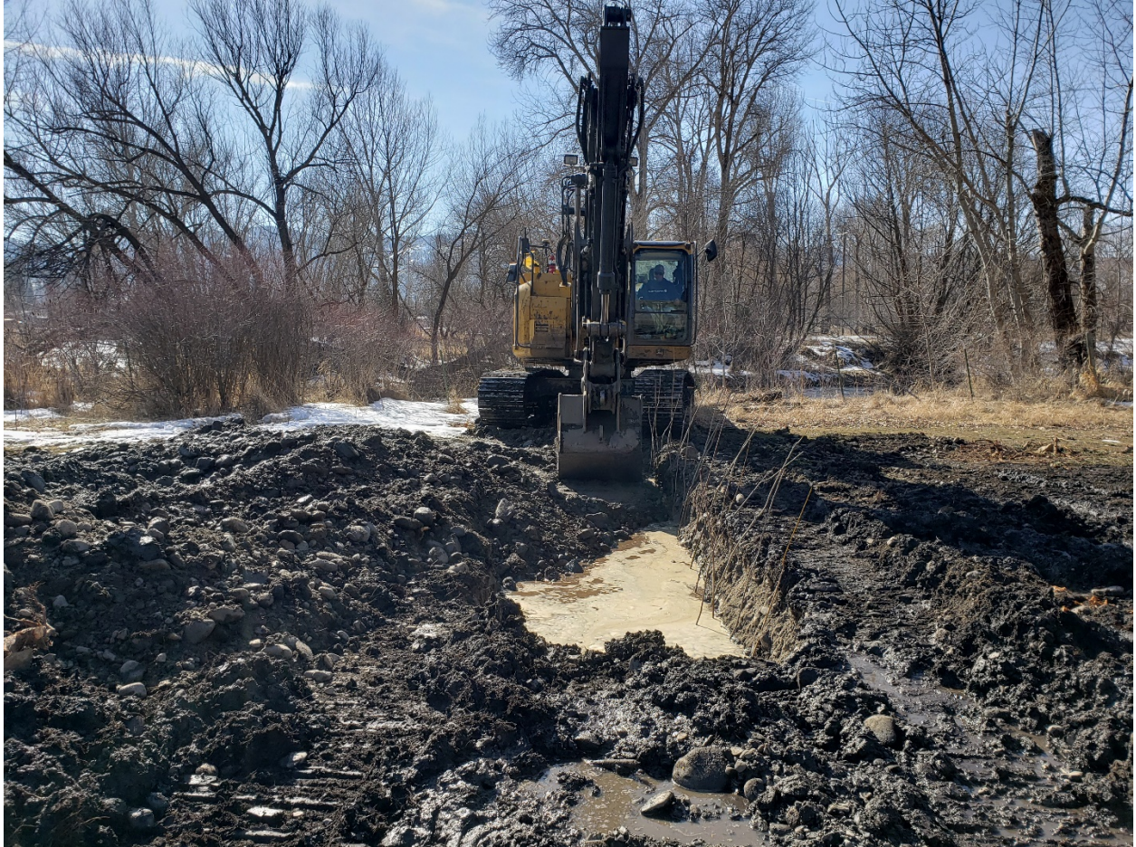
Figure 1. Willow trench installation along left/West bank of SC3, taken on 3/3.
