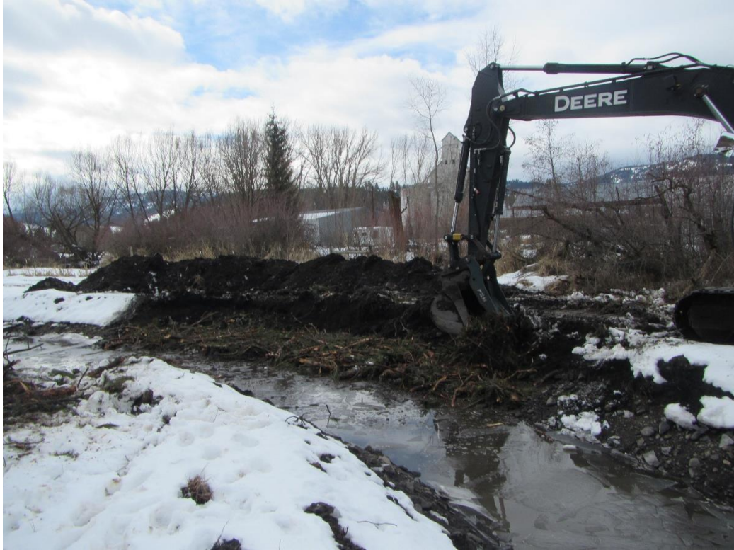
Figure 3. Brush Mattress install on SC3.
