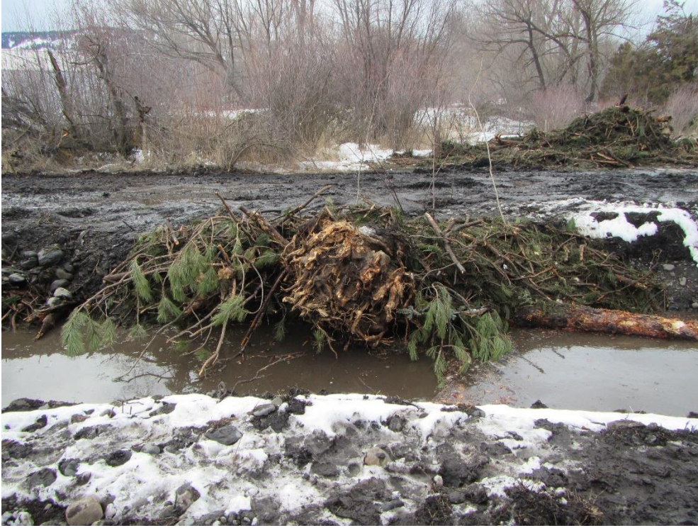
Figure 1. LWM installed at SC3 at ~Station 2+25.
