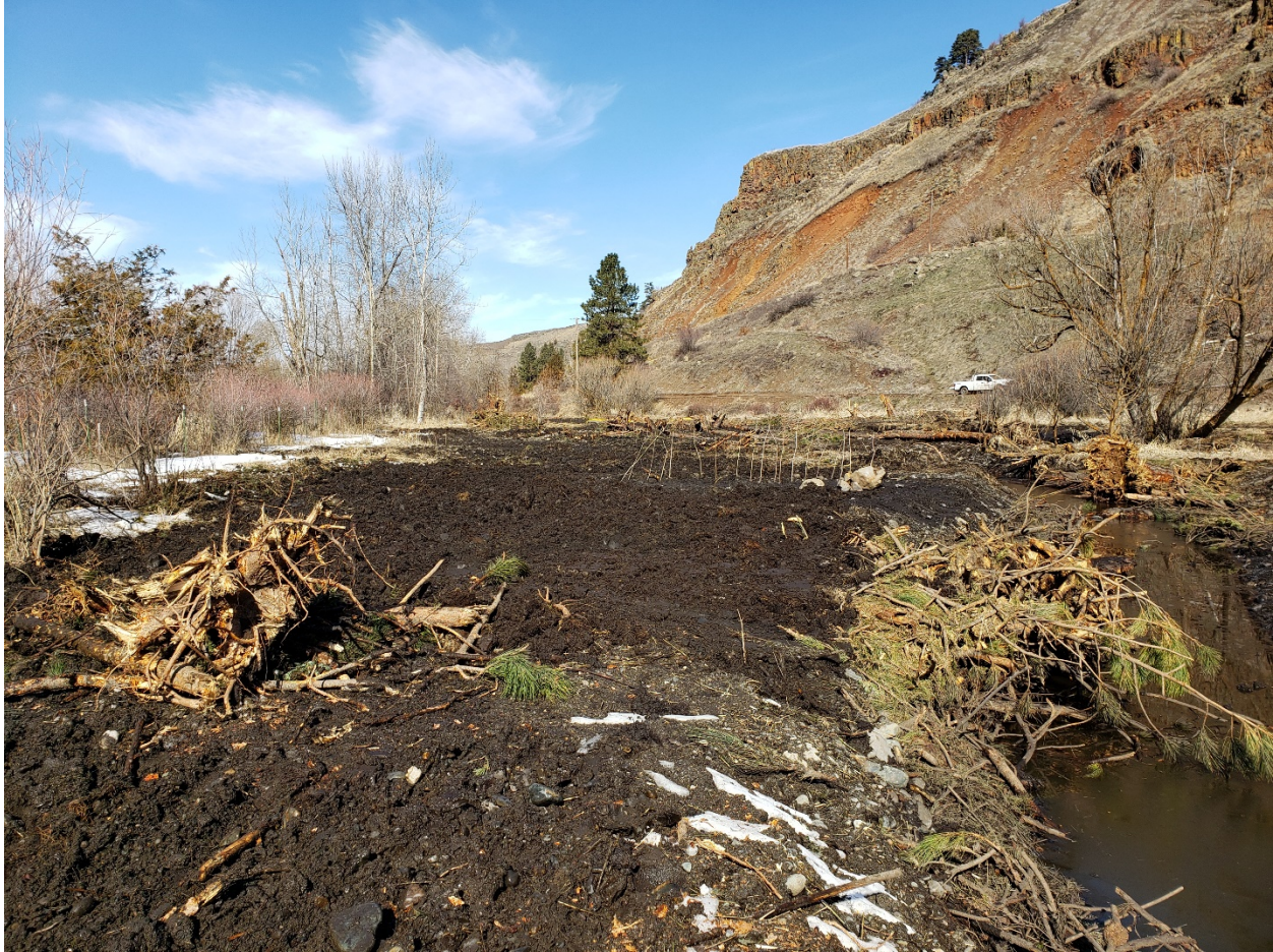
Figure 3. Completed floodplain roughness and willow trenches in West quadrant/left bank of SC3, taken 3/4.
