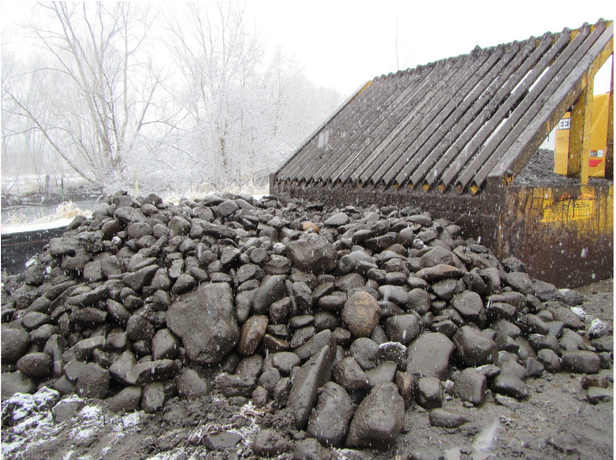
Figure 1. Sorted cobbles from SC3 fill. 4" rock sifter utilized.
