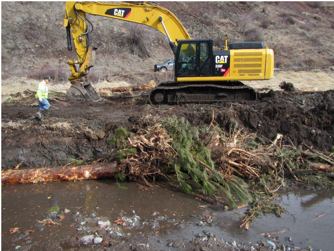
Figure 4. LWM install on Sc1 @ station 5+76
