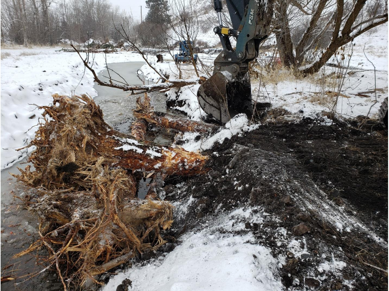
Figure 5. Installation of side channel whole tree habitat structure in SC3, taken 2/12.
