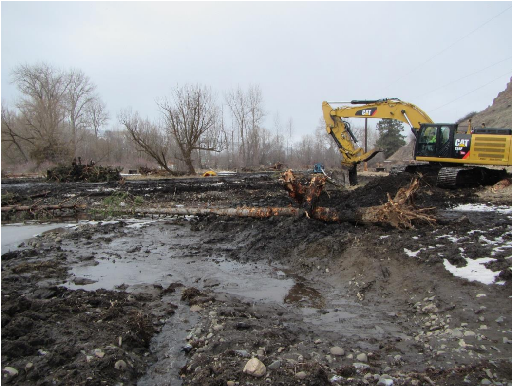
Figure 2. LWM installed at SC1 at ~Station 1+25.
