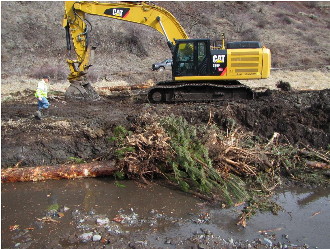
Figure 4. LWM install on Sc1 @ station 5+76
