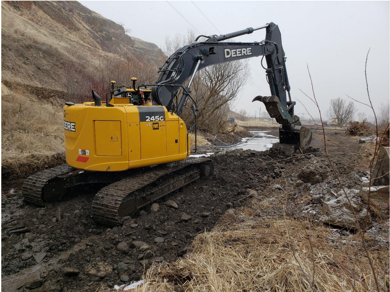
Figure 1. Riffle construction at downstream end of SC1, taken on 2/11.
