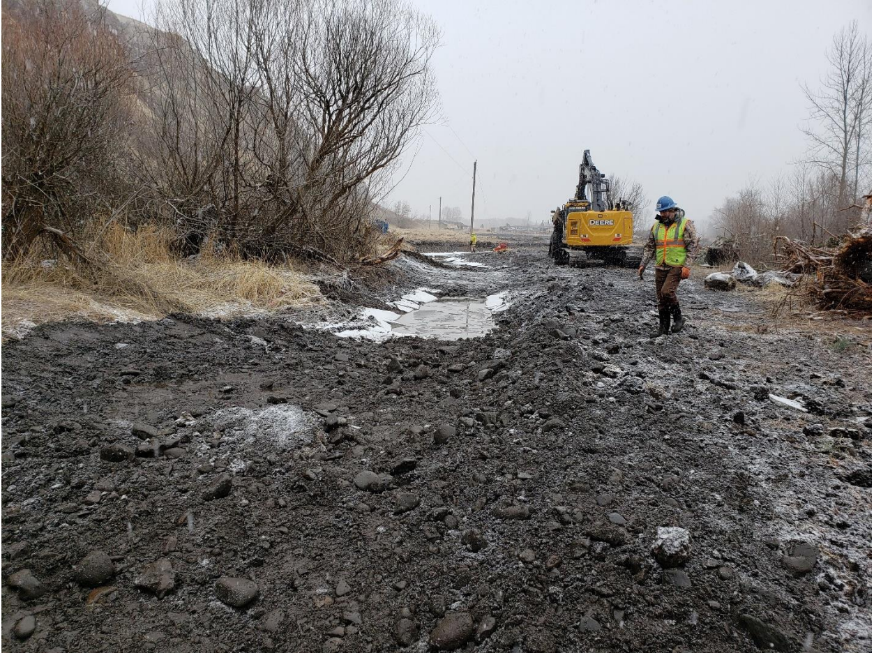
Figure 2. Riffle finished to grade in downstream end of SC1, taken on 2/11.
