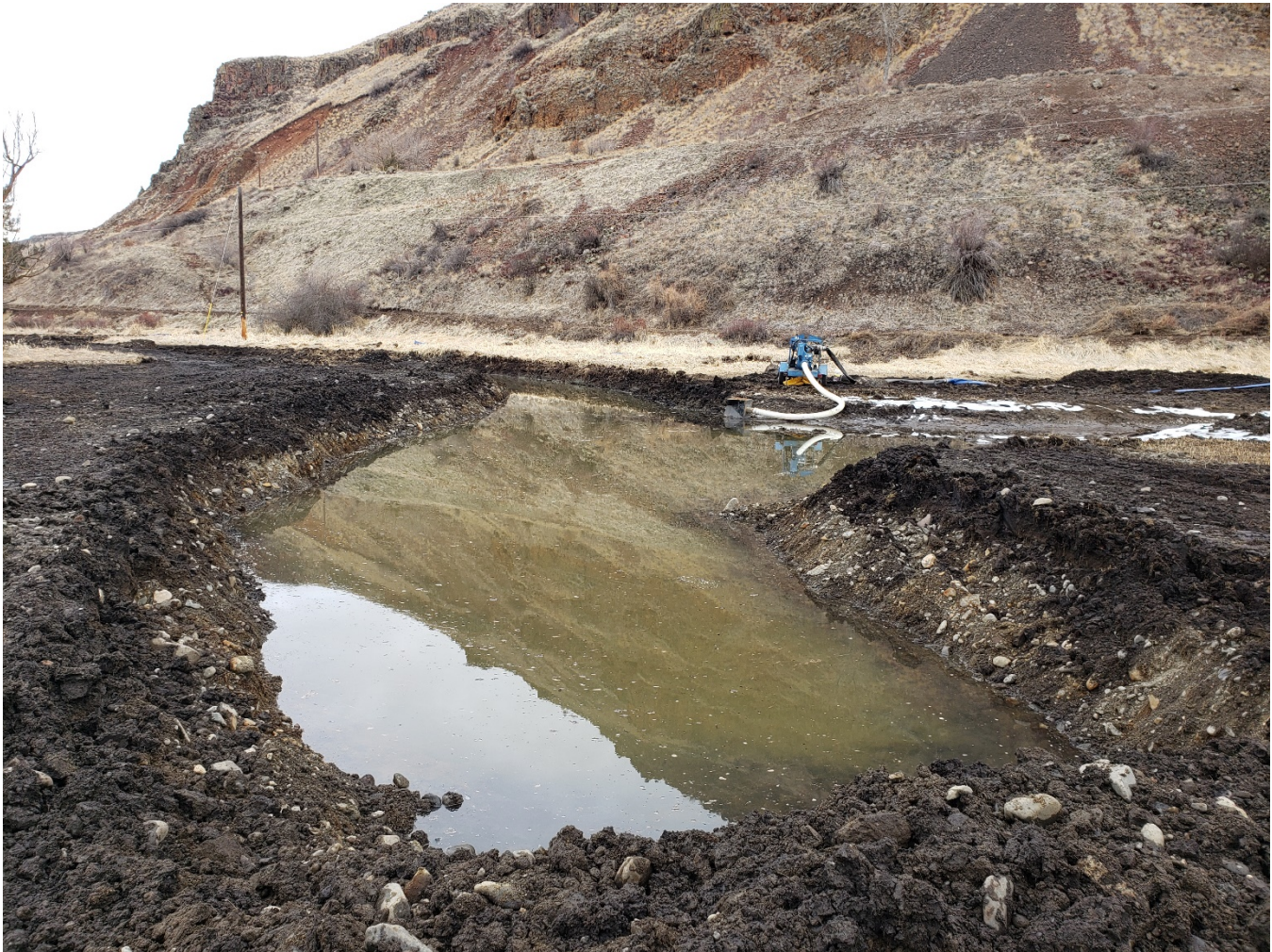
Figure 1. Fish screened pump and 6" hose pulling water out of side channel 1 below alcove node on 1/29/21.
