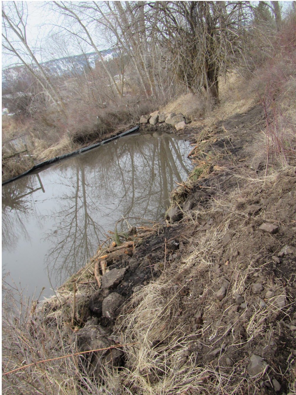
Figure 4. Silt fence placement between excavated alcove and earthen plug/river (3/8/21).
