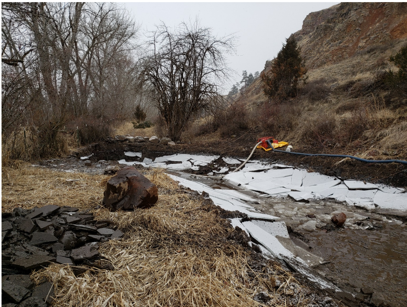
Figure 2. Fish screened pump and hose dewatering alcove area in side channel 1 and discharging pumped water upstream on the floodplain on 2/11/21.
