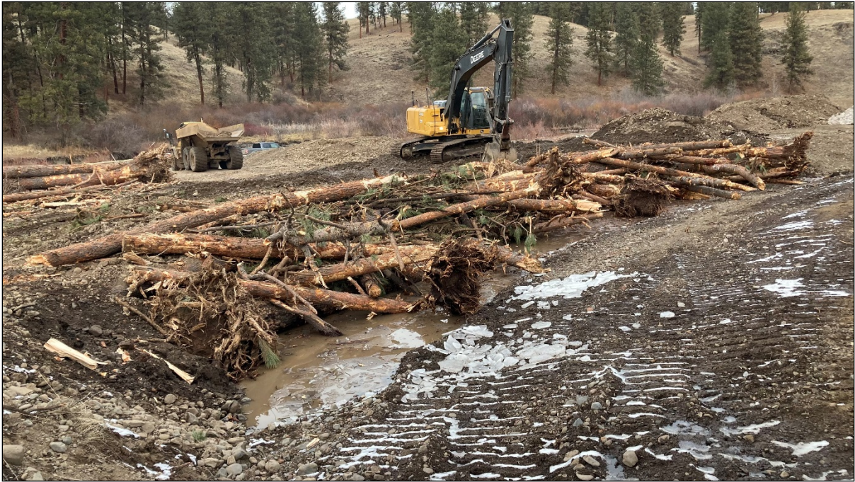
SIDE CHANNEL 5 POOL AND LARGE WOOD STRUCTURE
