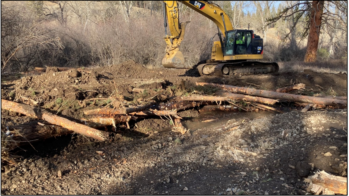
SIDE CHANNEL 5 CHANNEL GRADING
