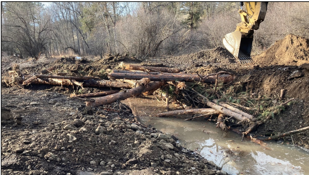
SIDE CHANNEL 5 POOL AND LARGE WOOD STRUCTURE
