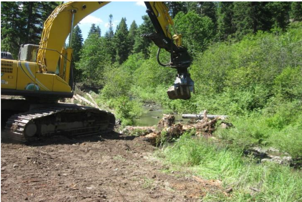
Placing Boulders on Structures
