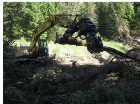
Moving trees w/shovel loader
