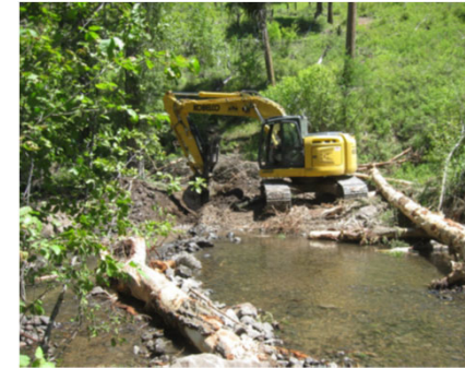
Excavator digging in rootwad
