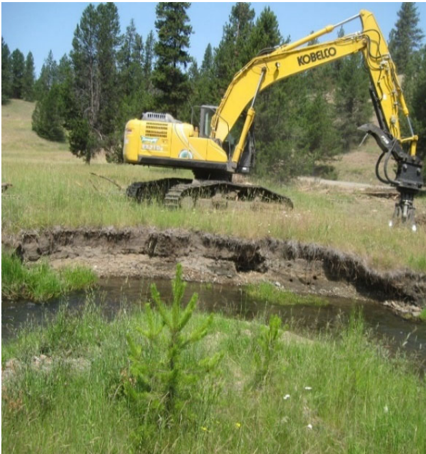
Shovel loader placing racking material into Limber Jim Creek
