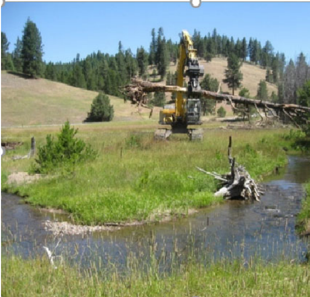
Shovel loader placing trees into Limber Jim Creek.
