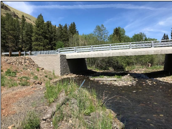
Photo 3: Top left: Standing upstream of culverts (2018). Culvert on the left is a flood relief culvert for times of high flow or when the two primary culverts are plugged. All 3 culverts will be removed and replaced with a bridge. Top right. New bridge without the need for overflow culverts (2019 and bottom left (2021).
