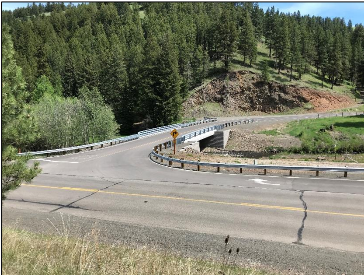
Photo 5: Top left: Standing across State Route 350 and looking east at former road alignment (2018). 4602 road skew was eliminated, a turn off lane from SR 350 was constructed, and the bridge was installed at the approximate center of the road curve. Top right: New road alignment and bridge (2019) and bottom left (2021).
