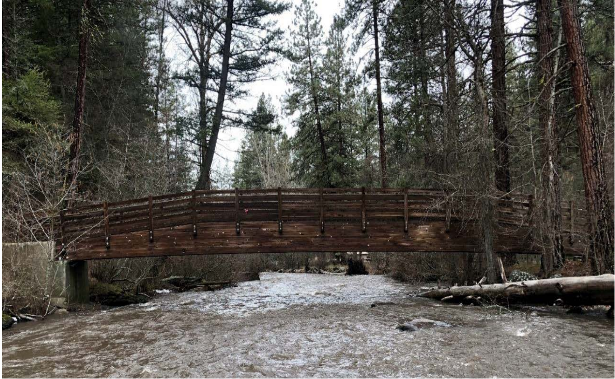
Pedestrian bridge and concrete abutments at Catherine Creek State Park, RM 48.6.
