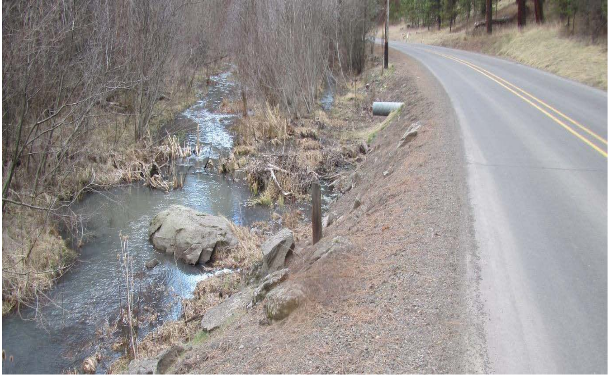
Historical Catherine Creek alignment at Catherine Creek State Park, located along the toe of the Highway 203 road prism.
