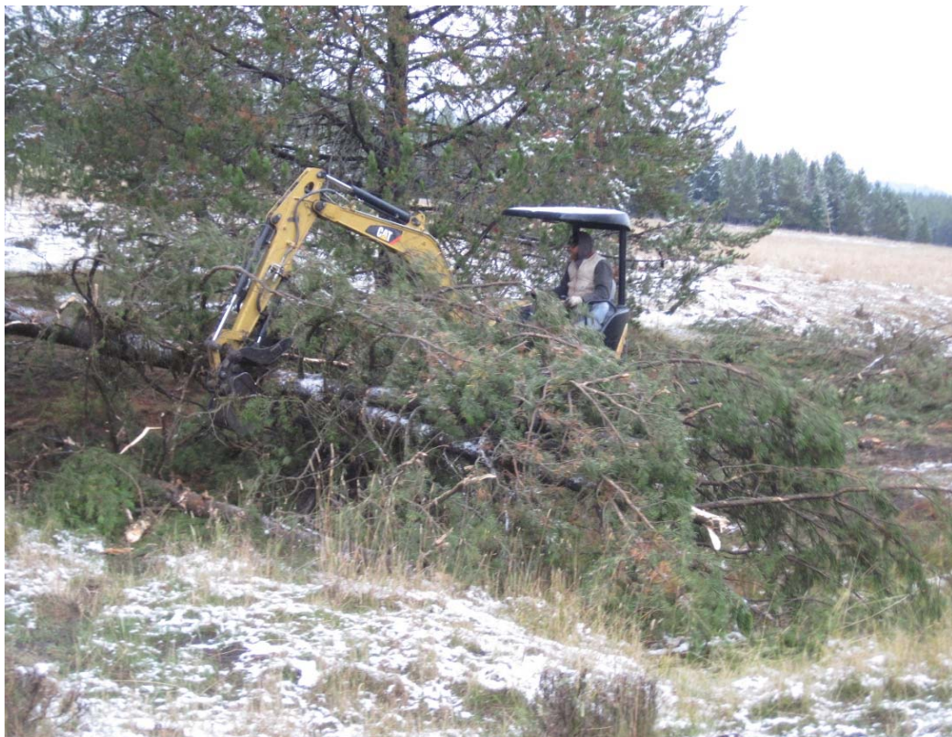
Mini excavator at work.
