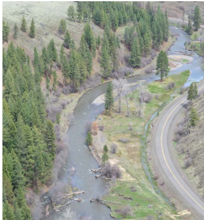
Figure 1 Existing Project Reach Condition
