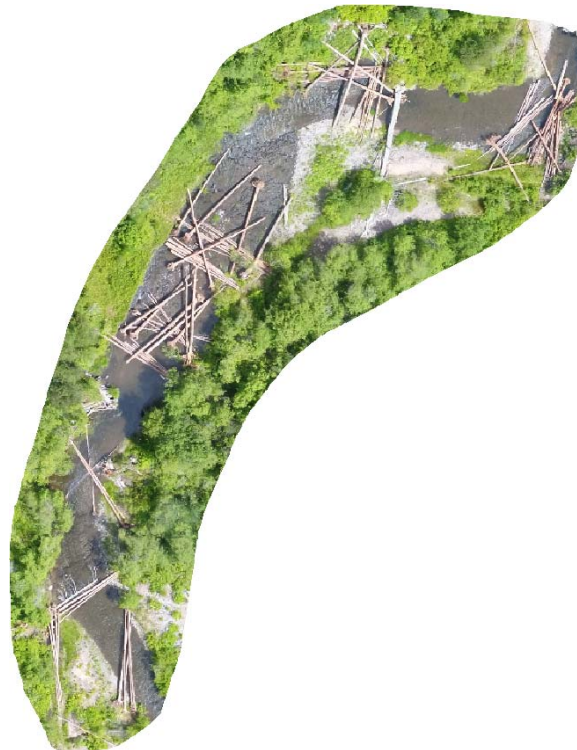
Figure 7 - Post Construction Drone Ortho Image
