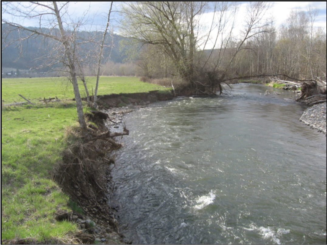
Figure 2. Looking downstream from the Baker property at the localized bank erosion (April 2007).
