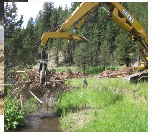
Placing racking material
