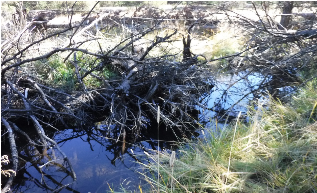
Log jam backed water into old structure on Chicken Creek
