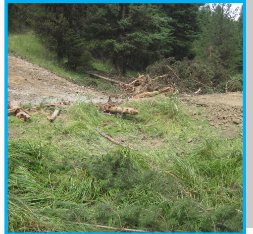
Removed culvert & constructed ford
