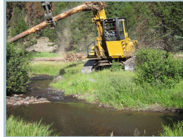
Placing wood with a log loader
