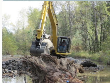
Placing rock for structure construction.
