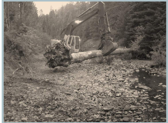
Fish Structure Construction.
