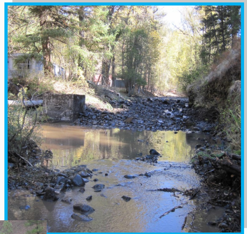
Post barrier removal.
