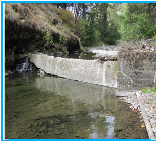
Barrier prior to removal.
