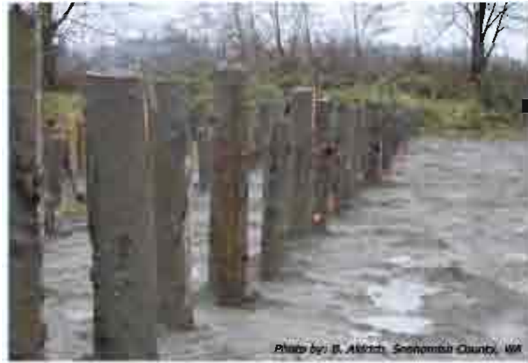
Example - Live Cottonwood Flood Fence (after first flood) (Note - Woven brush not added to this structure)
