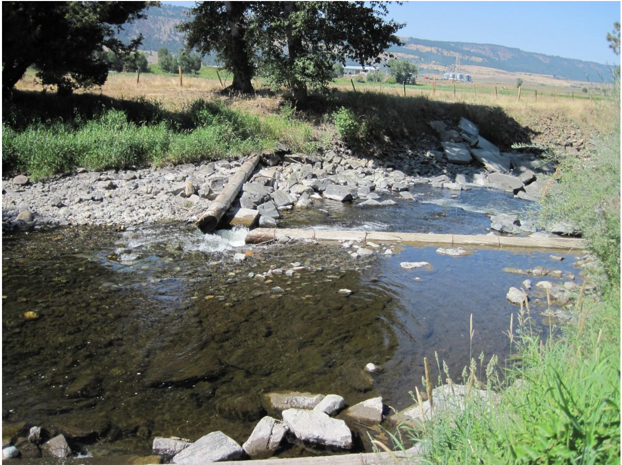
Photo 1: This photo was taken upstream of the second log weir just below the Tulley-Hill irrigation ditch diversion on the Lostine River, Wallowa County, OR. The photo was taken in late summer during low flow conditions on August 17, 2012. This is one of several rock and log weir structures that, at low flows, create jump height barriers to both upstream migrating juvenile fish, as well as adult Chinook migrating upstream to spawn.
