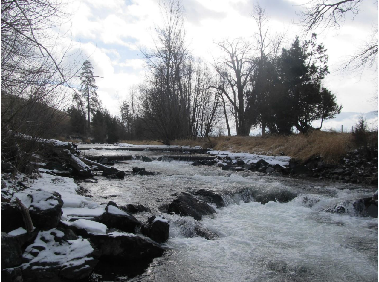
Photo 1: This photo was taken during the late fall downstream of all three step structures, below the Tulley-Hill irrigation diversion. The three barriers featured here include one rock weir (furthest downstream) and two log weirs. Fish passage issues arise over these structures at various flows, functioning as velocity barriers during high flows and jump height barriers during low flows.
